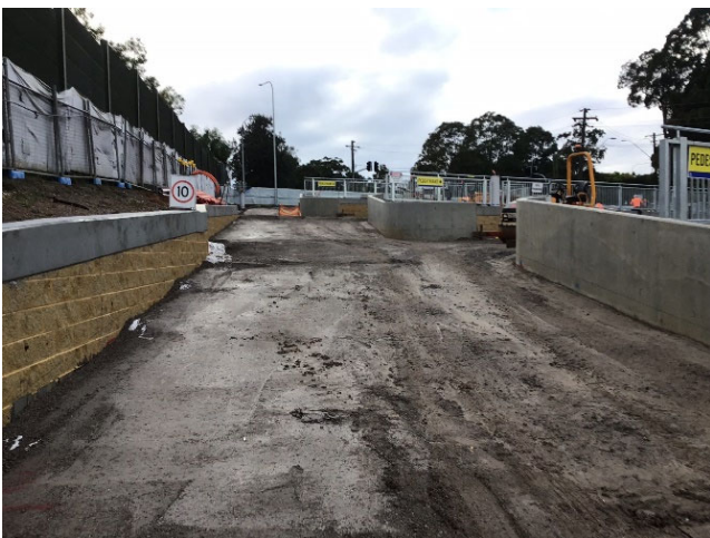
Work at North Rocks Commuter Car Park - July 2022
