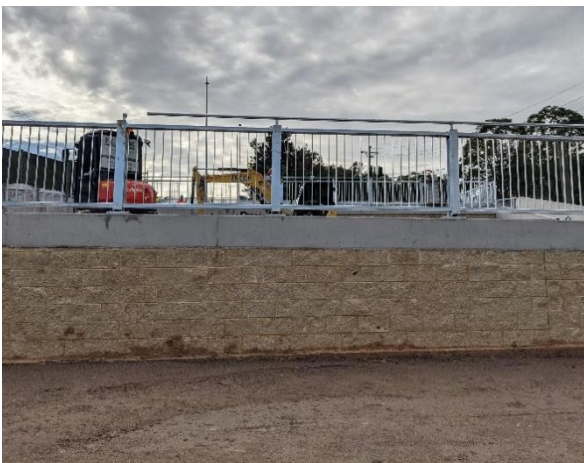
Completed retaining wall at North Rocks Commuter Car Park – May 2022
