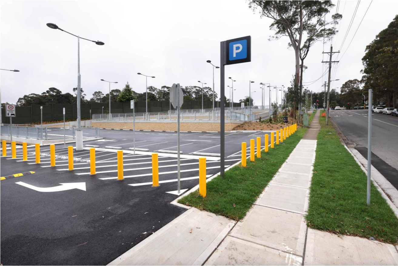
View of the completed North Rocks Commuter Car Park from Perry Street
