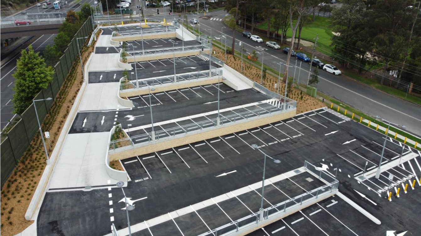
Aerial view of the completed North Rocks Commuter Car Park
