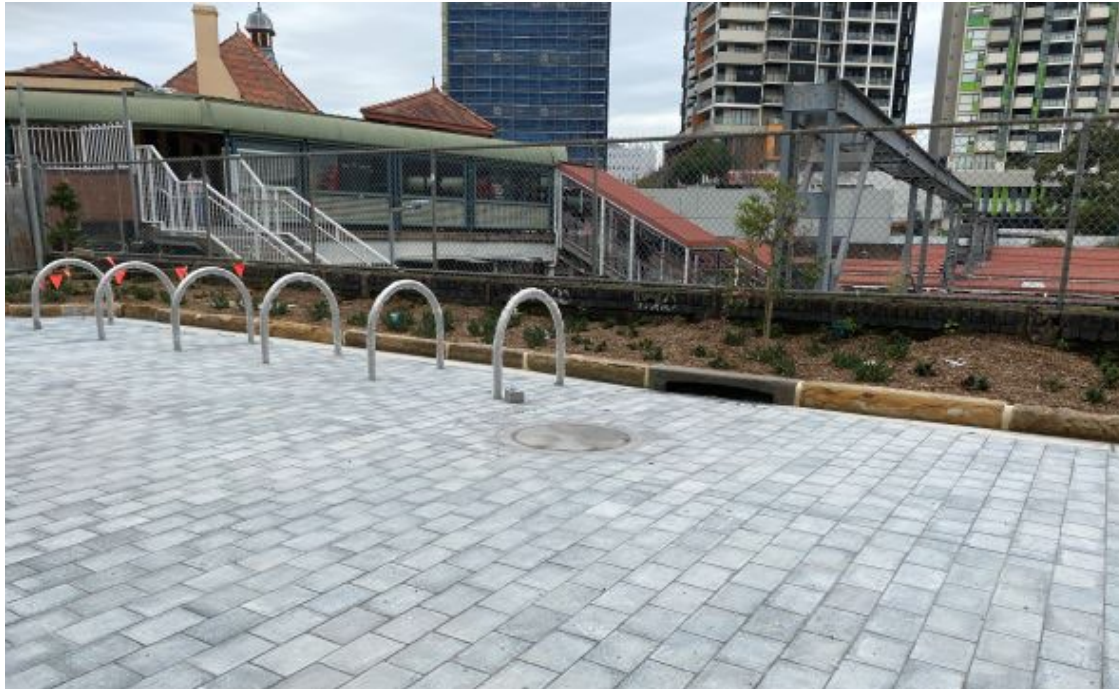
Image above shows new paved area in stage one of the Little Eveleigh Street shared zone
