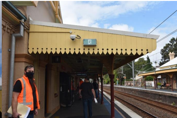
Figure 39. Decorative timber valance to the awning ends (Source: Artefact, 2021)
