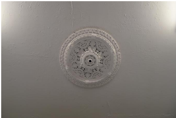
Figure 48. Original plaster ceiling with decorative plaster ceiling rose to the small waiting room (Source: Artefact, 2021)
