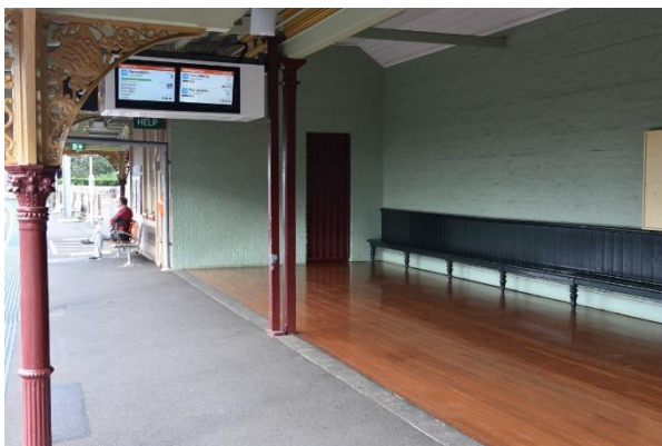
Figure 62. Platform 3 waiting room, features original timber floorboards, painted brick walls and timber bench seating (Source: Artefact, 2021)
