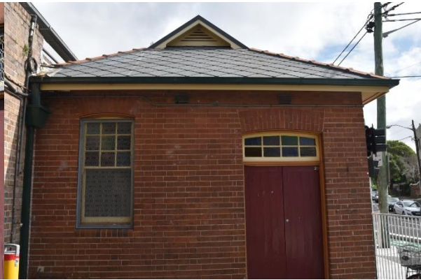
Figure 71. Original diamond pattern fibre cement roof tiles in a slate finish with terracotta ridges. Half gable features timber barge board and timber ventilation slats (Source: Artefact, 2021)
