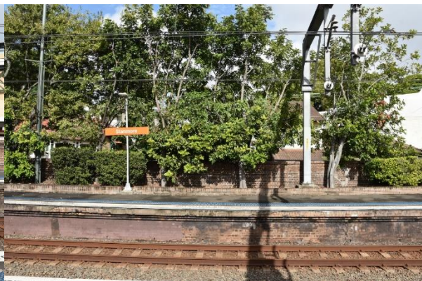
Figure 85. Brick retaining wall, hedging and trees on platform 3. Areas of the platform retaining wall have been rendered and painted, evidence of repair or replacement (Source: Artefact, 2021)
