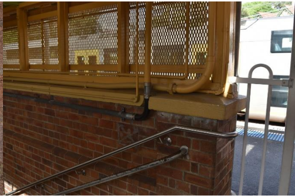
Figure 105. Metal mesh to clerestory windows, brick wall with rendered cement coping (Source: Artefact, 2021)
