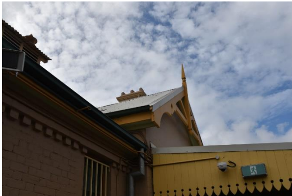
Figure 38. Original decorative timber barge board and finial details to gable end (Source: Artefact, 2021)
