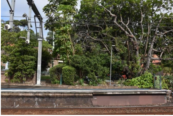
Figure 88. Concrete platform extension to the western end of the platform (Source: Artefact, 2021)
