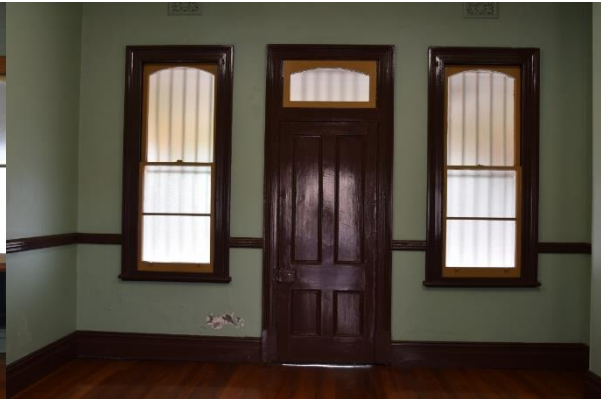
Figure 47. Interior of smaller waiting room, features painted rendered masonry walls, timber dado, high profiled timber skirting, original timber architraves and window and door joinery, and timber floorboards (Source: Artefact, 2021)
