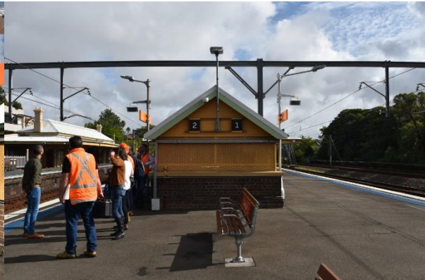
Figure 75. Platform 1/2 subway lantern as viewed from gable end, metal mesh to clerestory windows, brick plinth (Source: Artefact, 2021)
