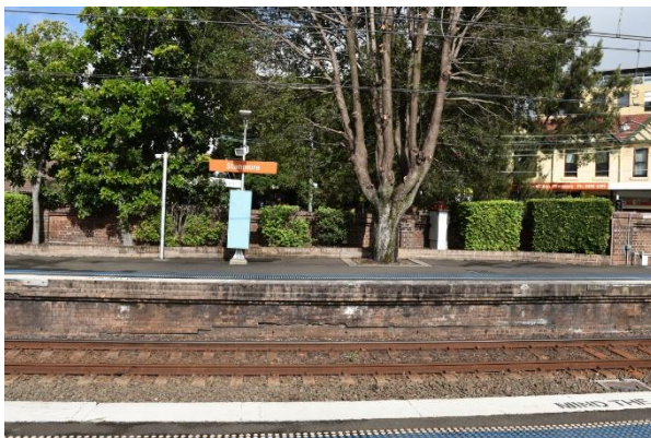
Figure 84. English bond brick retaining wall and brick coping used to construct platform 3 visible from platform 2 (Source: Artefact, 2021)
