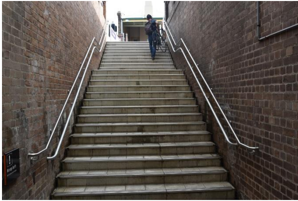
Figure 108. Concrete tile lined stairs to Platform 3. Original handrail retained beneath compliant contemporary handrail (Source: Artefact, 2021)
