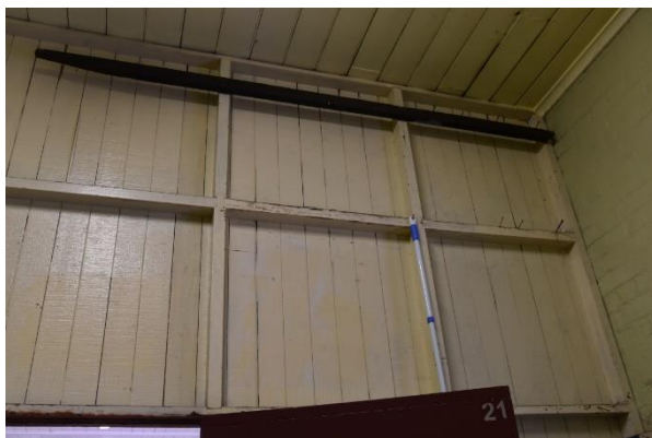
Figure 52. Original timber partition and timber boarded ceiling in the store room (Source: Artefact, 2021)
