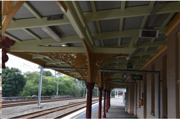
Figure 41. Original cast iron columns and decorative filigree brackets with the 'NSWGR' insignia (Source: Artefact, 2021)
