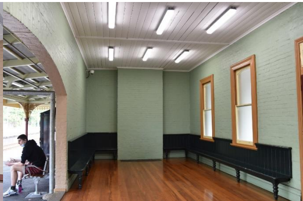
Figure 45. Interior of the large waiting room, features original timber boarded ceilings, painted brick walls with painted original high profiled timber skirting, and timber floorboards (Source: Artefact, 2021)
