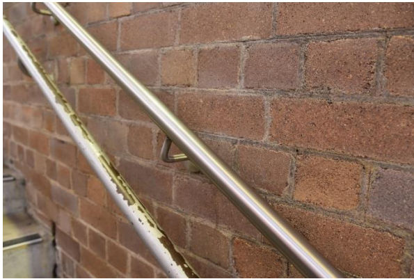
Figure 104. Original handrail retained beneath contemporary to code handrail (Source: Artefact, 2021)
