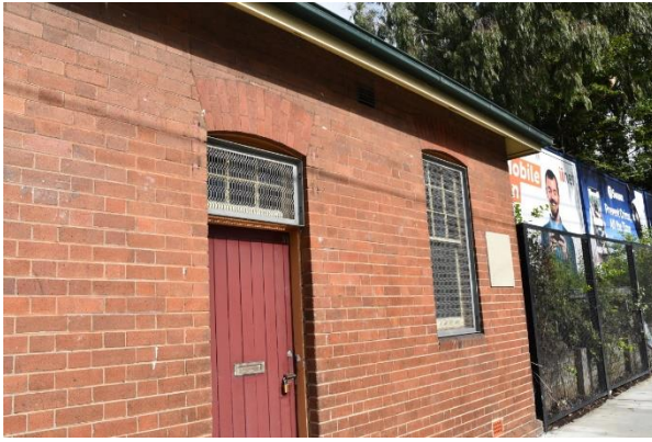
Figure 68. Flemish bond brick walls, brick voussoirs above original timber boarded door with highlight window and multipaned double hung timber sash windows (Source: Artefact, 2021)
