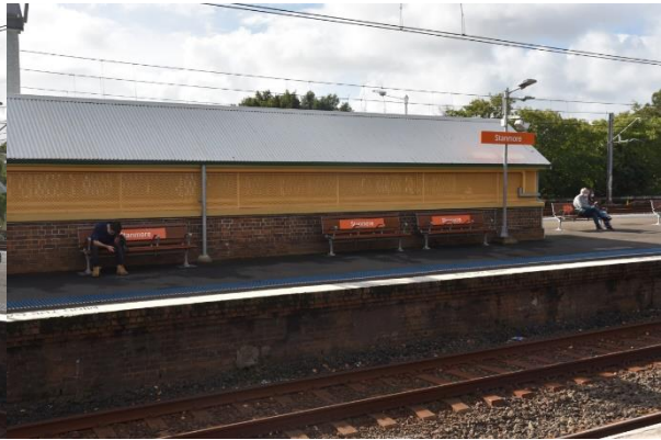
Figure 83. English bond brick retaining walls and brick coping to construct platform 1/2 as visible from platform 3 (Source: Artefact, 2021)
