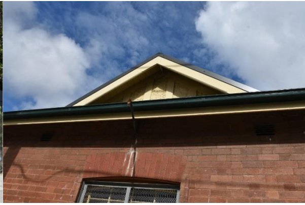
Figure 69. Half gable, with cement fibre and timber cladding (Source: Artefact, 2021)
