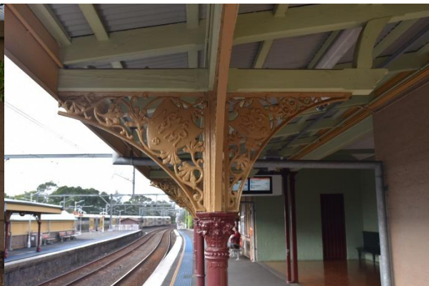
Figure 61. Decorative cast iron awning columns and filigree brackets. Brackets include 'NSWGR' insignia, their tapered ends have been cut off when the awning was foreshortened (Source: Artefact, 2021)
