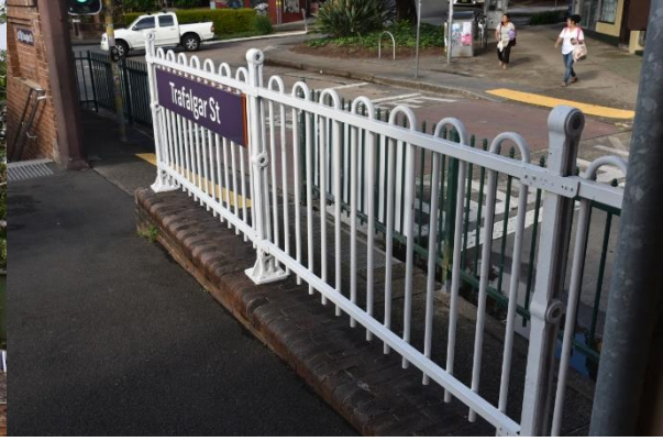
Figure 89. Trafalgar Street entry to platform 3, original dwarf brick wall, with non-original steel loop top fencing (Source: Artefact, 2021)
