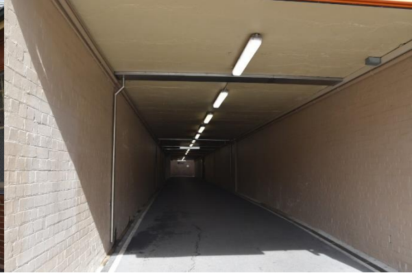
Figure 97. Pedestrian subway as you enter from Douglas Street, painted brick walls, concrete ceiling and asphalt floor (Source: Artefact, 2021)
