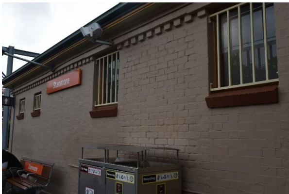
Figure 42. Dentilled stringcourse detail to building (Source: Artefact, 2021)
