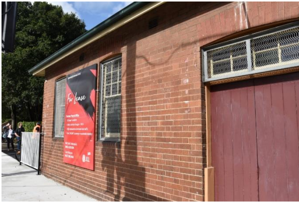
Figure 70. Original timber boarded double entry doors at centre of Douglas Street façade (Source: Artefact, 2021)
