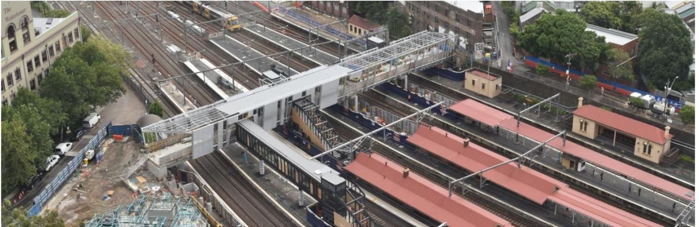
In February, we installed lifts, stairs and sections of roofing across platforms 4 to 9 on the bridge. We are now half way through installing the new lifts, which is an exciting milestone as it's one of many steps to improving accessibility at Redfern Station. We thank the community for their patience and understanding while we carried out this important work.
