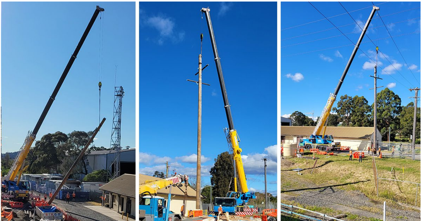
Pictured: High voltage power poles being relocated for the new footbridge construction to continue.
