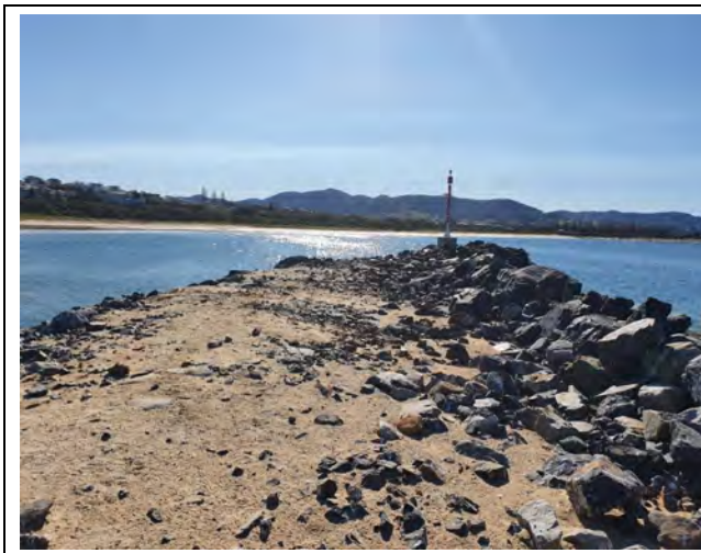
Boat ramp breakwater to the north
