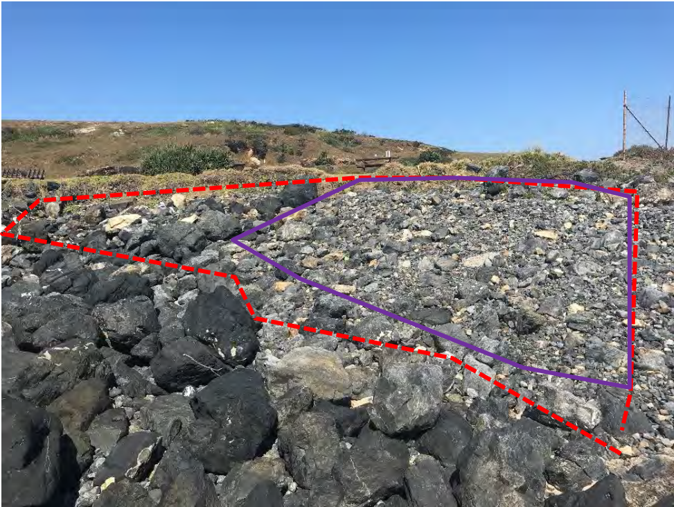
Figure 23: Clear transition between very small core material (purple) exposed and some scattered underlayer. Foreground shows “Floating” larger armour remaining (outside red dashed line).
