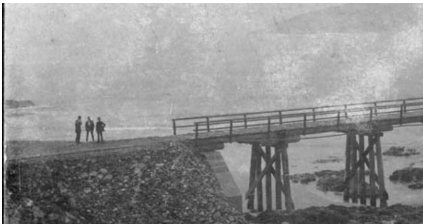
Plate 6: "Viaduct to South Coffs Island 1915". Completed (Source: Coffs Harbour Library: "Picture Coffs Harbour" bookmark link: https://coffsharbour.spydus.com/cgi-bin/spydus.exe/ENQ/WPIC/BIBENQ?SETLVL=&BRN=199681 )
