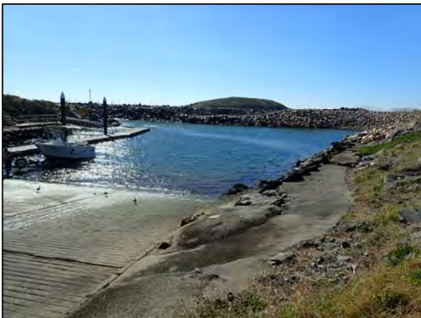
Figure 3.5 Boat ramp facing north east
