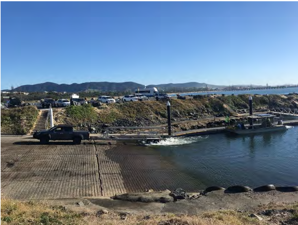
Figure 11: Coffs Harbour Boat Ramp and Pontoon, showing user “dry” launching, utilising the existing western pontoon
