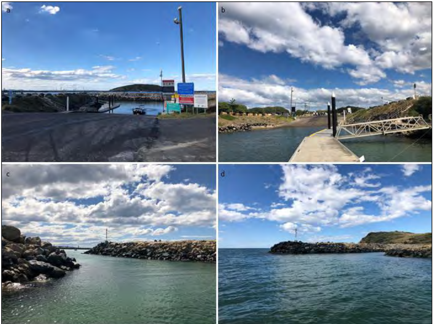
Plate 1: Existing boat ramp, pontoons, seawalls and breakwater.
