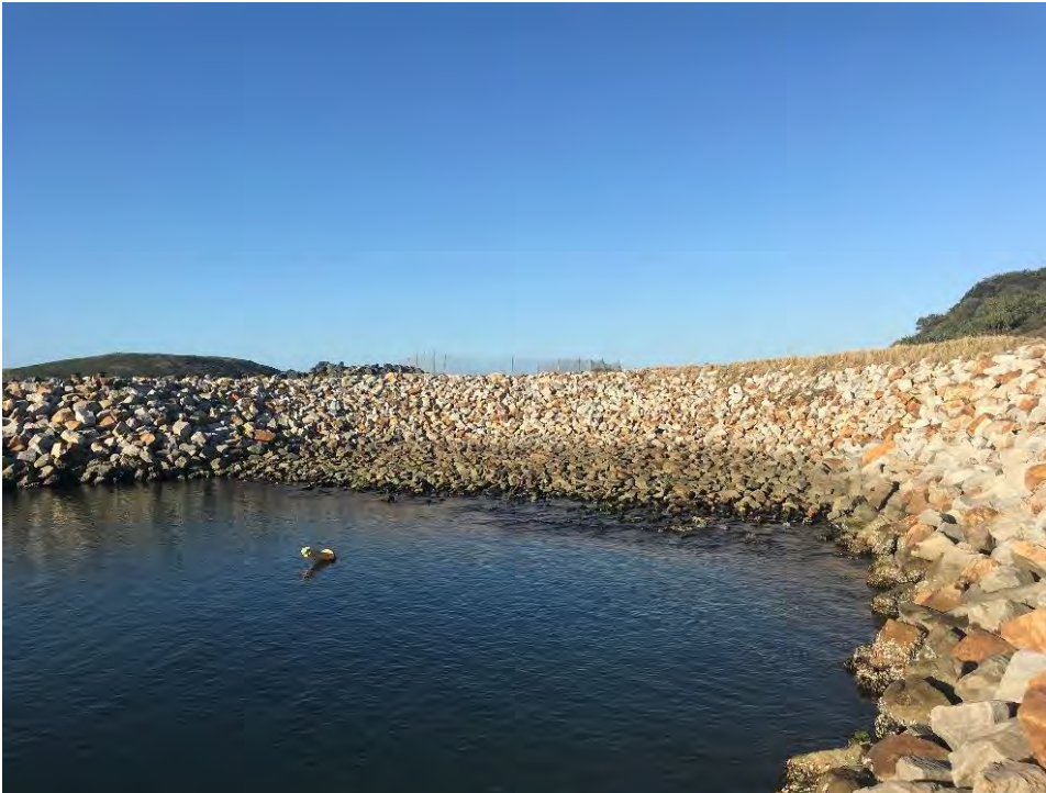
Figure 12: Photo of the Boat Ramp Basin extension constructed in 2015 to dissipate Seiching energy
