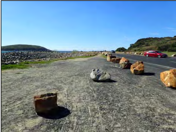
Figure 3.6 CP4 western end facing east
