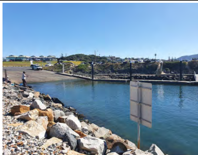
Existing boat ramp, facing south -west
