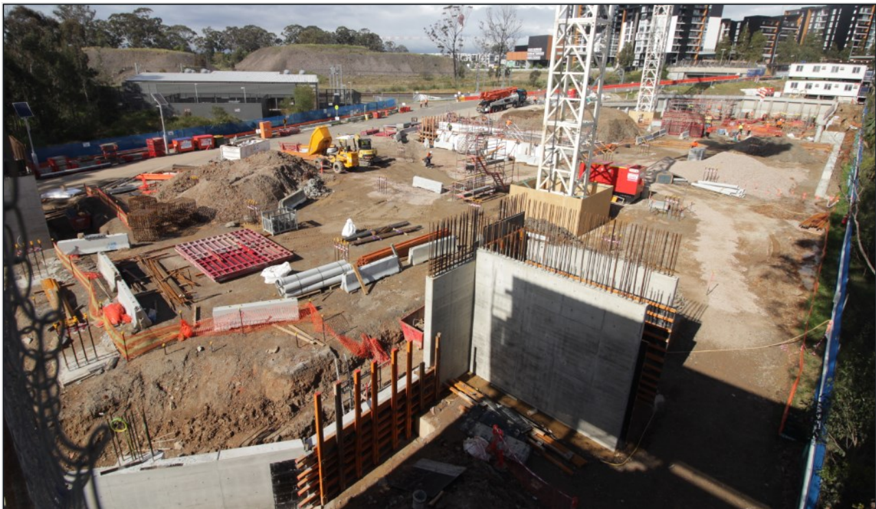
Construction progress on the Edmondson Park North Commuter Car Park.
