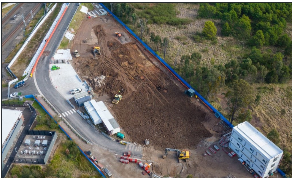
Construction progress on the Edmondson Park North Commuter Car Park project.
