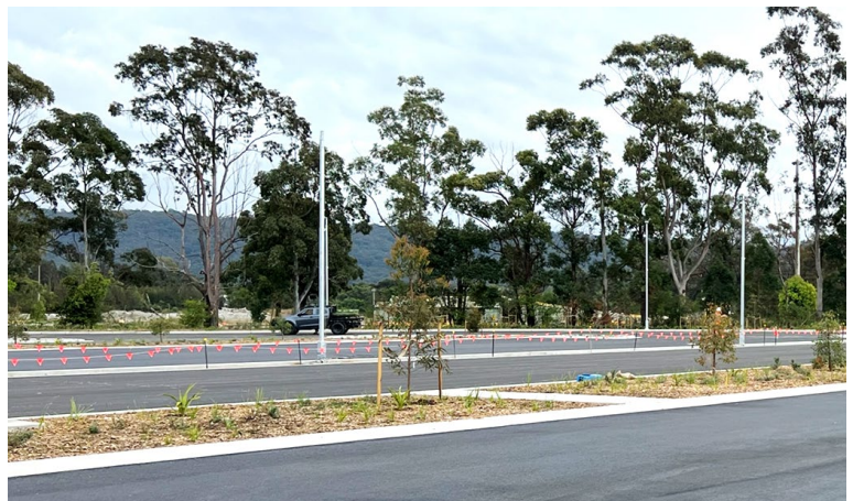
Picture above – asphalting and landscaping are progressing
