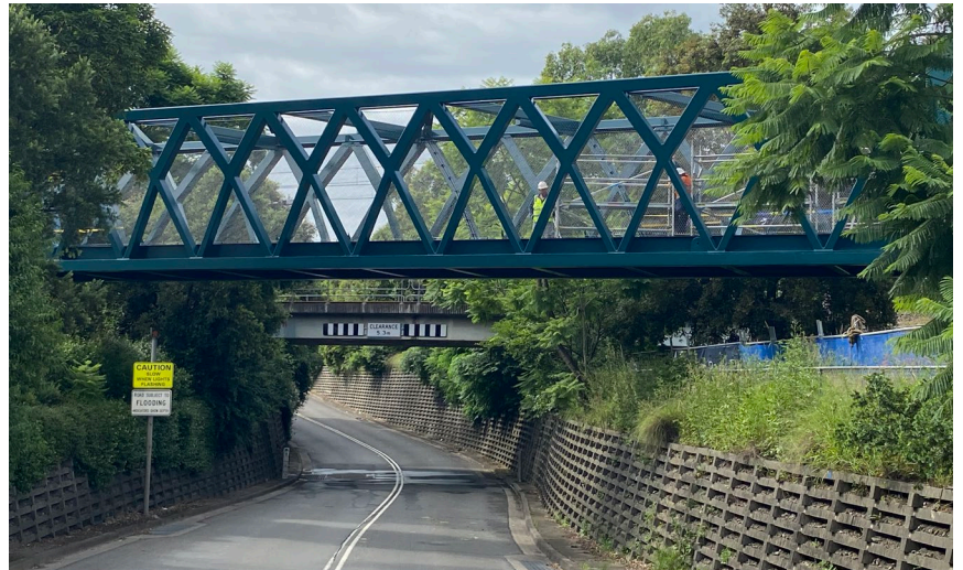
Photo above: the footbridge across Old Bathurst Road now in place
