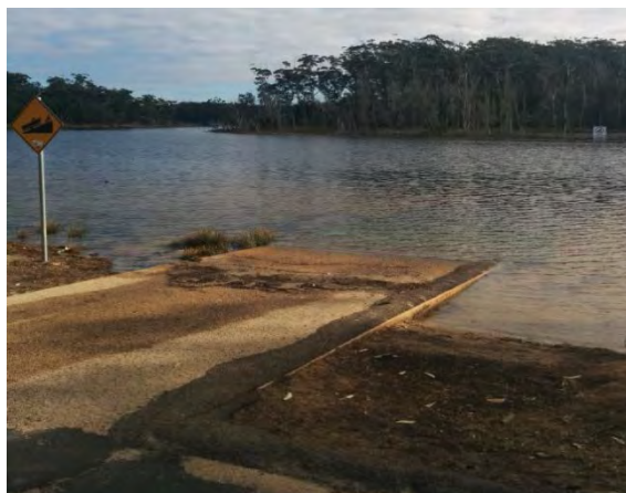
Narrow access at Durras Lake boat ramp
