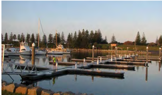
Marina pontoons being installed at Bermagui
