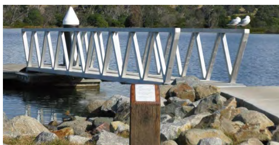
Mogareeka Boat Ramp Pontoon
