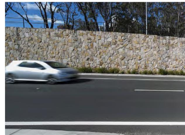
Figure 3.20 Informal pattern of a sandstone clad retaining wall along the Great Western Highway.
