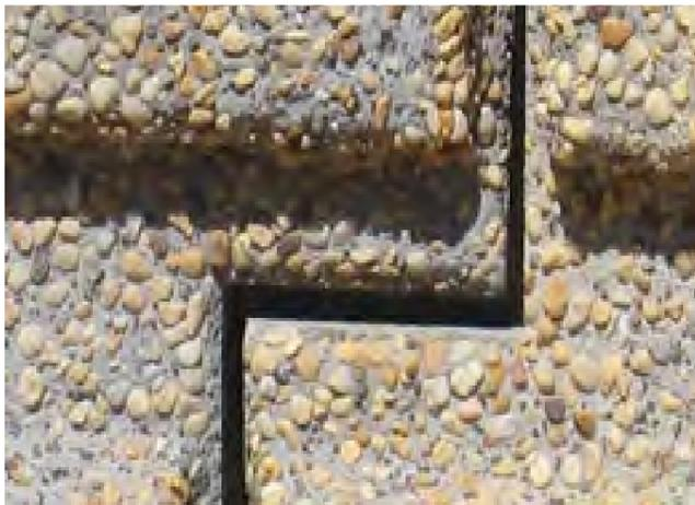
Figure 3.24 Exposed aggregate was used for the retaining walls facing Katoomba Showground. Careful detailing and material selection are important urban design considerations. Photo credit: Catherine Dung.
