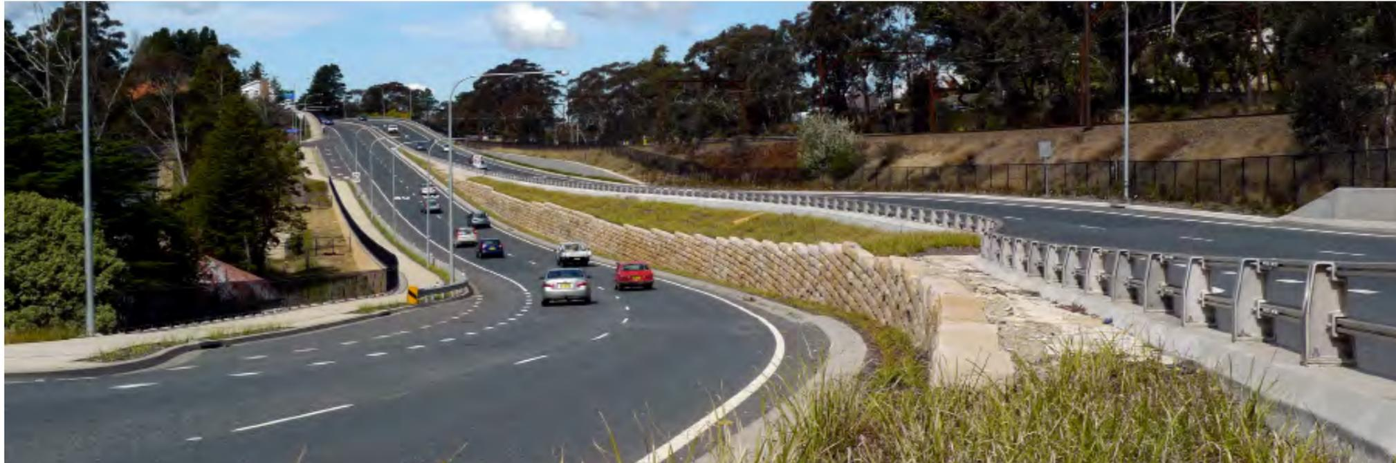
Figure 3.22 Vertically split carriageways along the Great Western Highway near Leura. The wall helps integrate the road with the topography and articulates the scale of the road. The median retaining wall has been constructed from sandstone blocks salvaged from a pre-existing heritage wall, demonstrating a sensitive design response to the setting. Photo credit: Catherine Dung.
