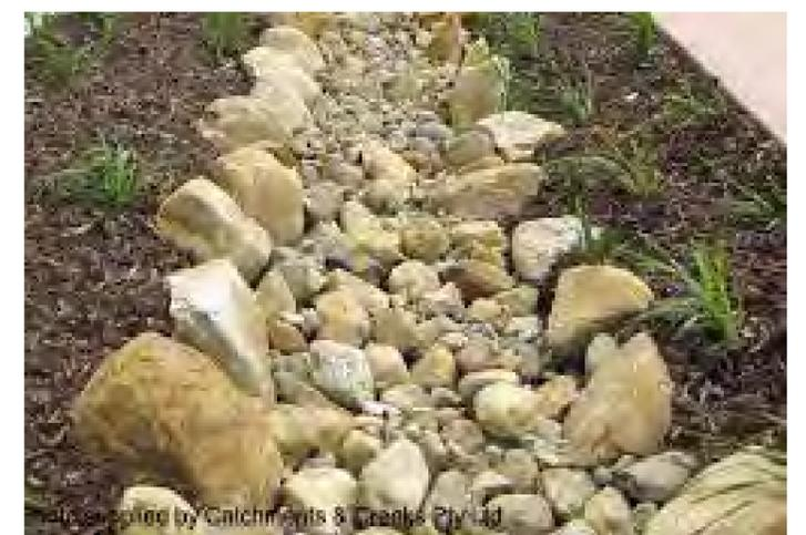
Figure 3.16 Use of sandstone rock in swales limits the visual exposure of concrete drains.
