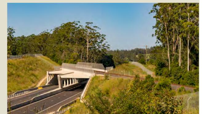
Figure 4.25 Example of a railway and highway bridge interface with a strong skew. Pacific Highway at Warrell Creek
