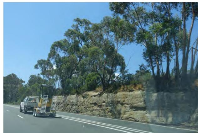
Figure 4.4 Where small rock cuttings occur, leave this exposed with no vegetation strip in front. This expresses the existing situation and maximises retention of trees
