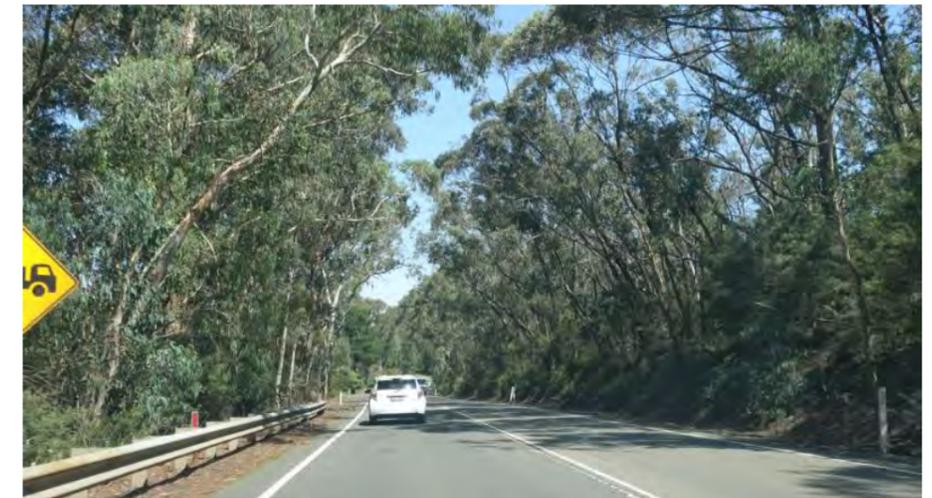
Figure 3.10 Barriers can maximise retention of existing trees close to road pavement edge- the overlapping canopies reinforce the natural bushland setting
