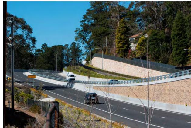
Figure 4.20 The careful integration of retaining walls can articulate their scales and express the topography. Sympathetic materials should be used for these elements facing the road or community
