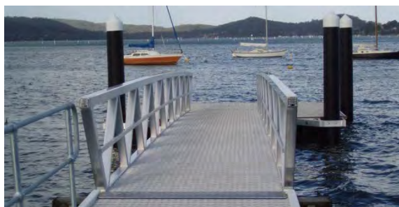
Couche Park Wharf & Pontoon, Brisbane Water
