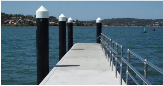
Booragul Jetty Replacement
