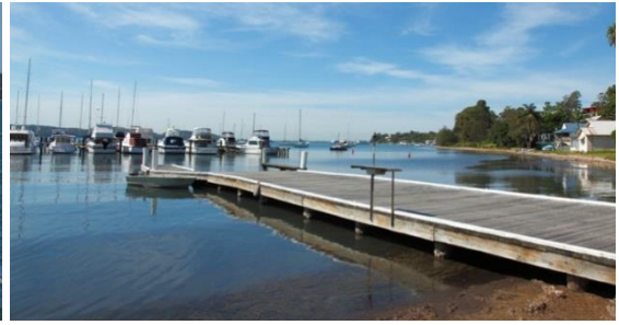
RMYC Boat Launching ramp upgrade
