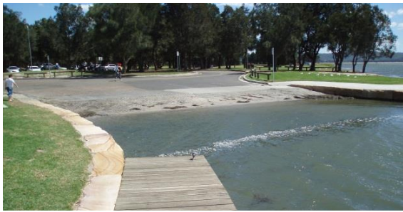
Picnic Point Boat Ramp and Facilities Upgrade
