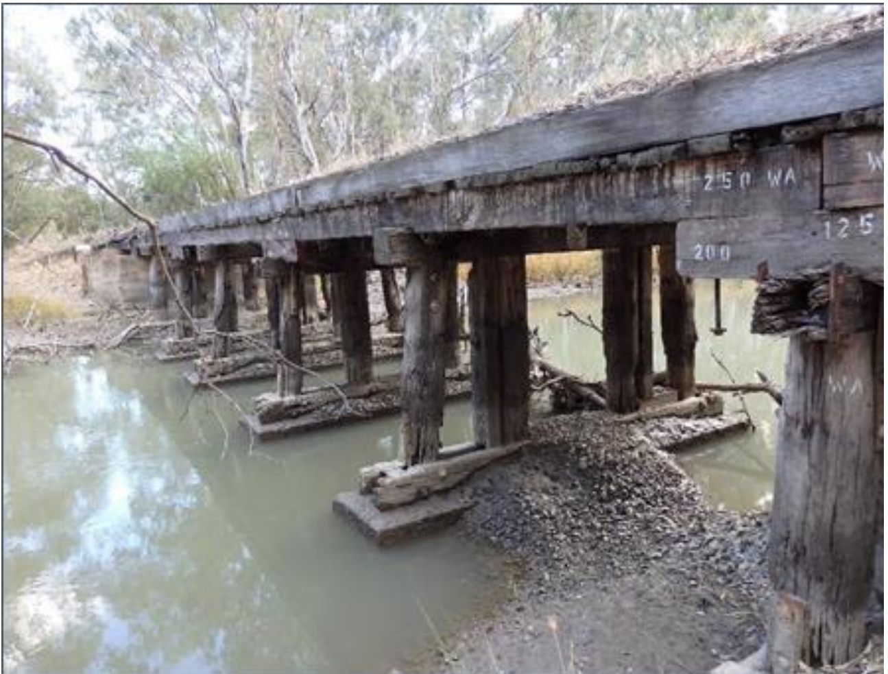
Figure 6 - Underbridge over Morundah Creek, Morundah
