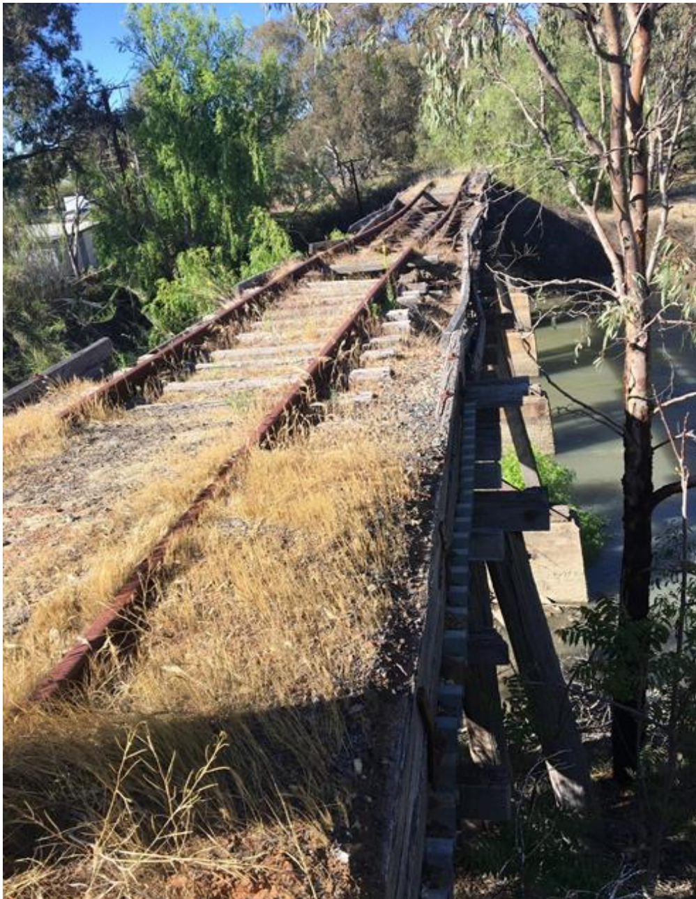
Figure 4 – Typical Timber Ballast Deck Structure
