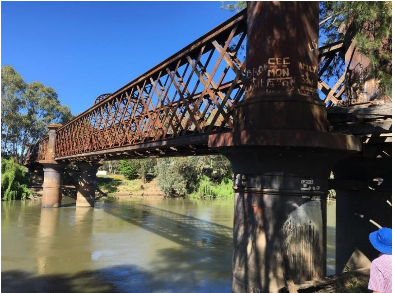
Figure 1 – Narrandera Truss Bridge across the Murrumbidgee
