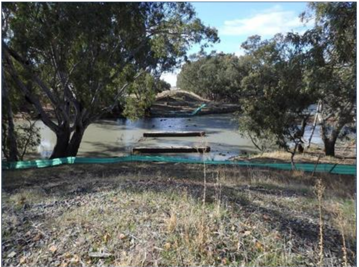
Figure 3 - Removed Underbridge over Billabong Creek, Jerilderie
