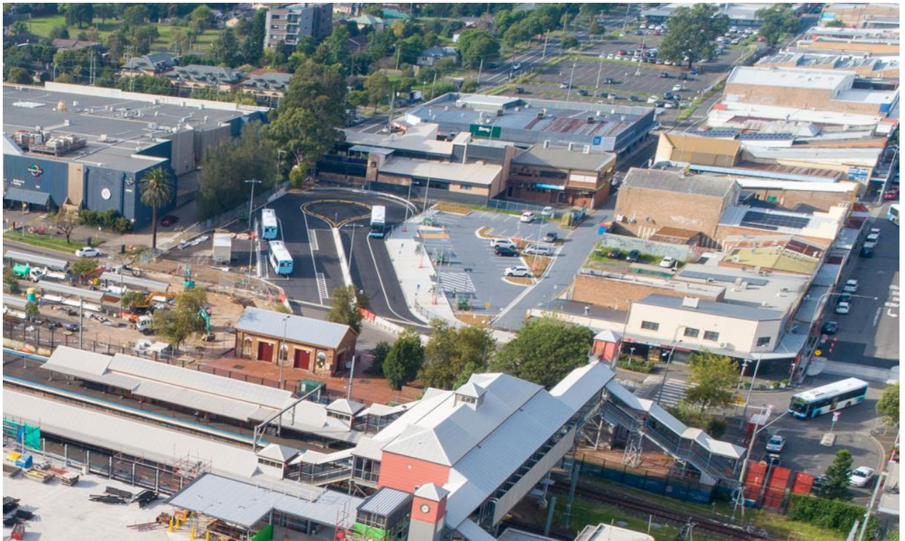
Aerial view of the completed temporary bus interchange at St Marys
