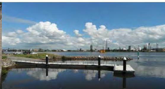
North Stockton Boatramp Pontoon
