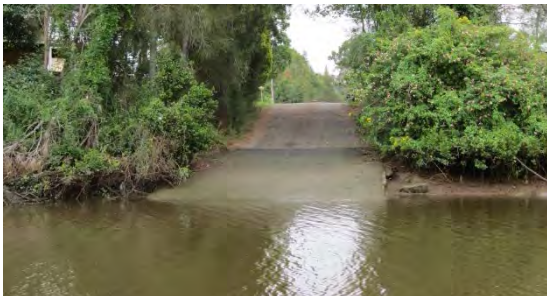
Single lane boat ramp with no infrastructure for temporary boat tie up to assist in launching and retrieval
