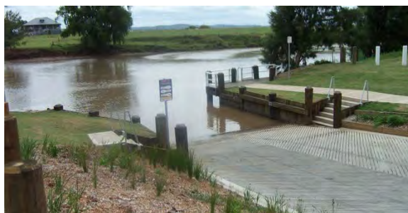
Morpeth Boat Ramp Upgrade –Queens Wharf
