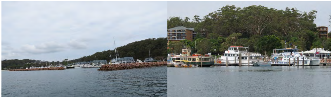
Entrance to the Anchorage Marina at Corlette
