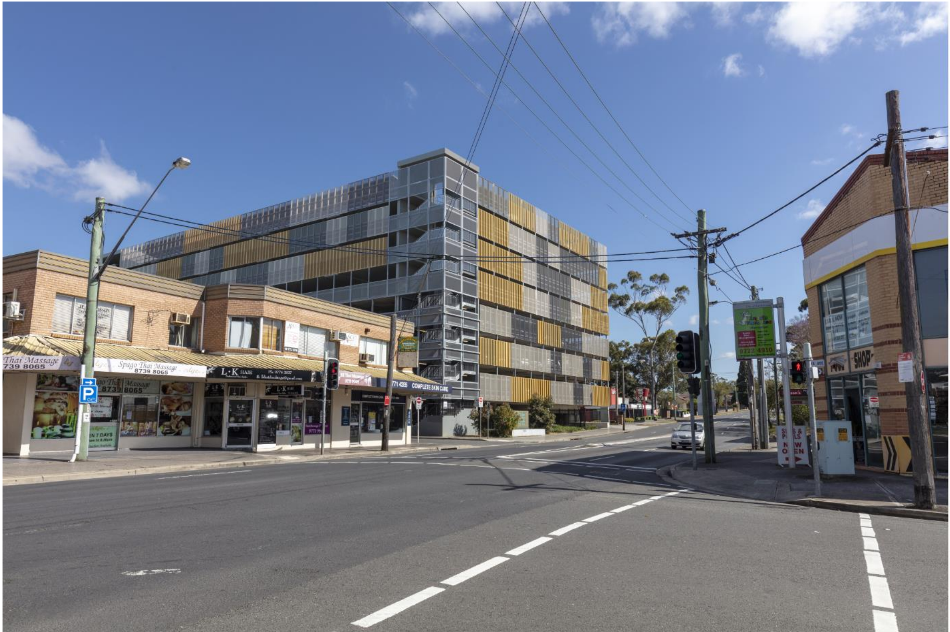
Figure 3-4 Photomontage of proposed commuter car park looking from The River Road, facing north-west. Indicative only and subject to detailed design.
