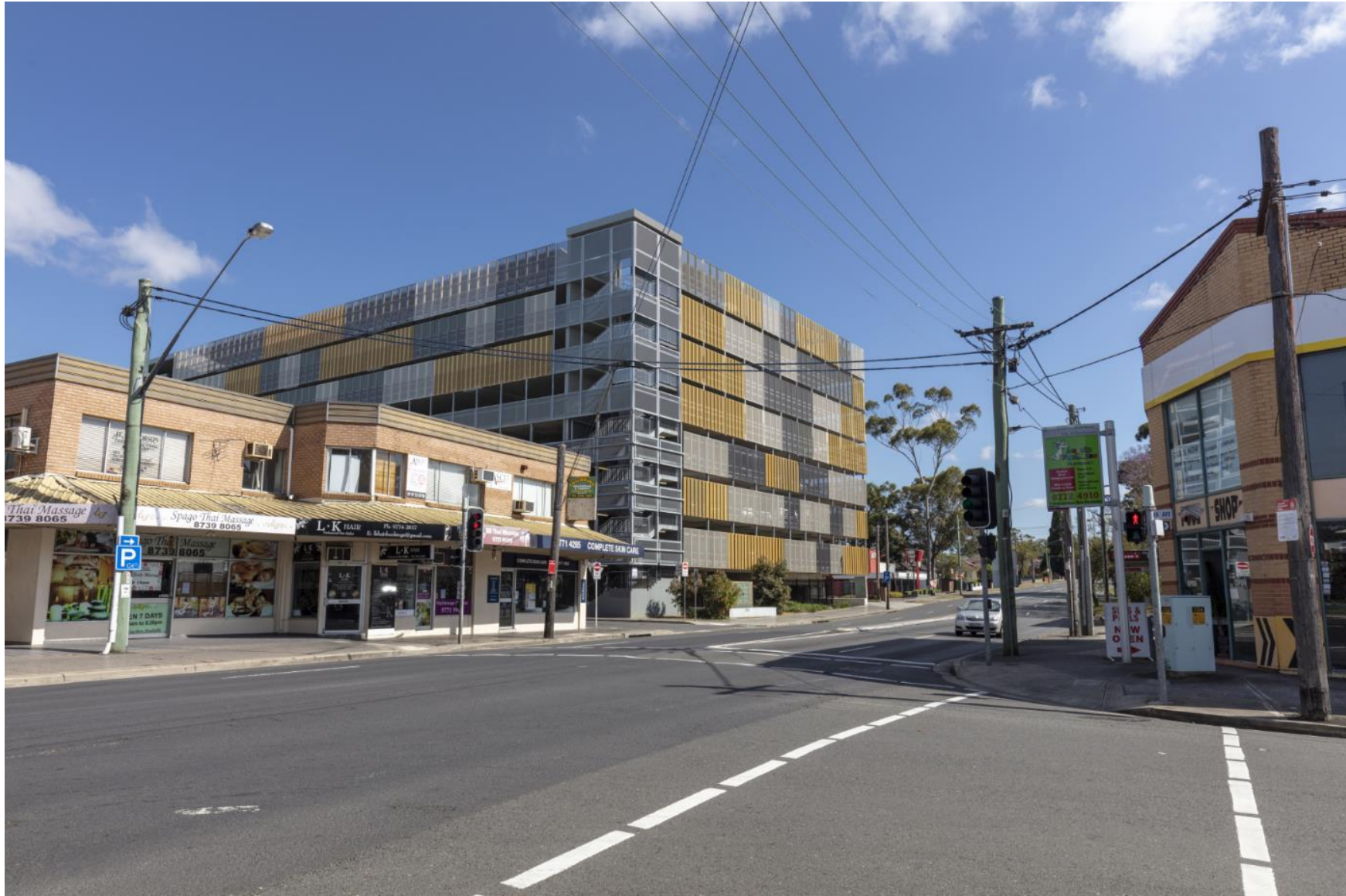
Figure ES-2 Artist's Impression of the Proposed Revesby Commuter Car Park Expansion (indicative only, subject to detailed design)
