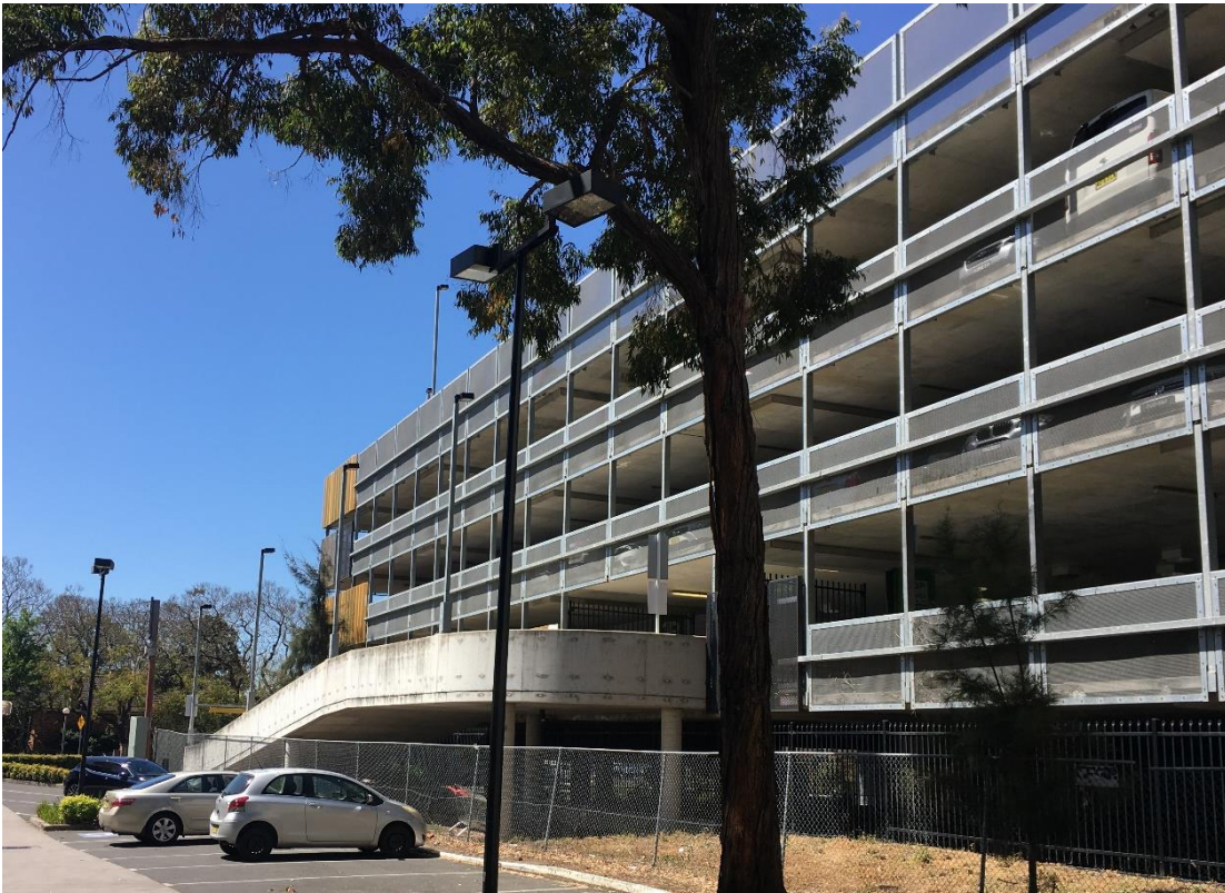
Figure 1-5 The existing car park looking east towards The River Road
