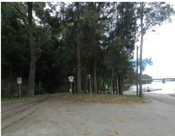
Approach to Greys Beach boat ramp. Orientation restricts efficient use of ramp.
