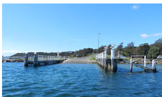
Crookhaven Heads Boat Ramp
