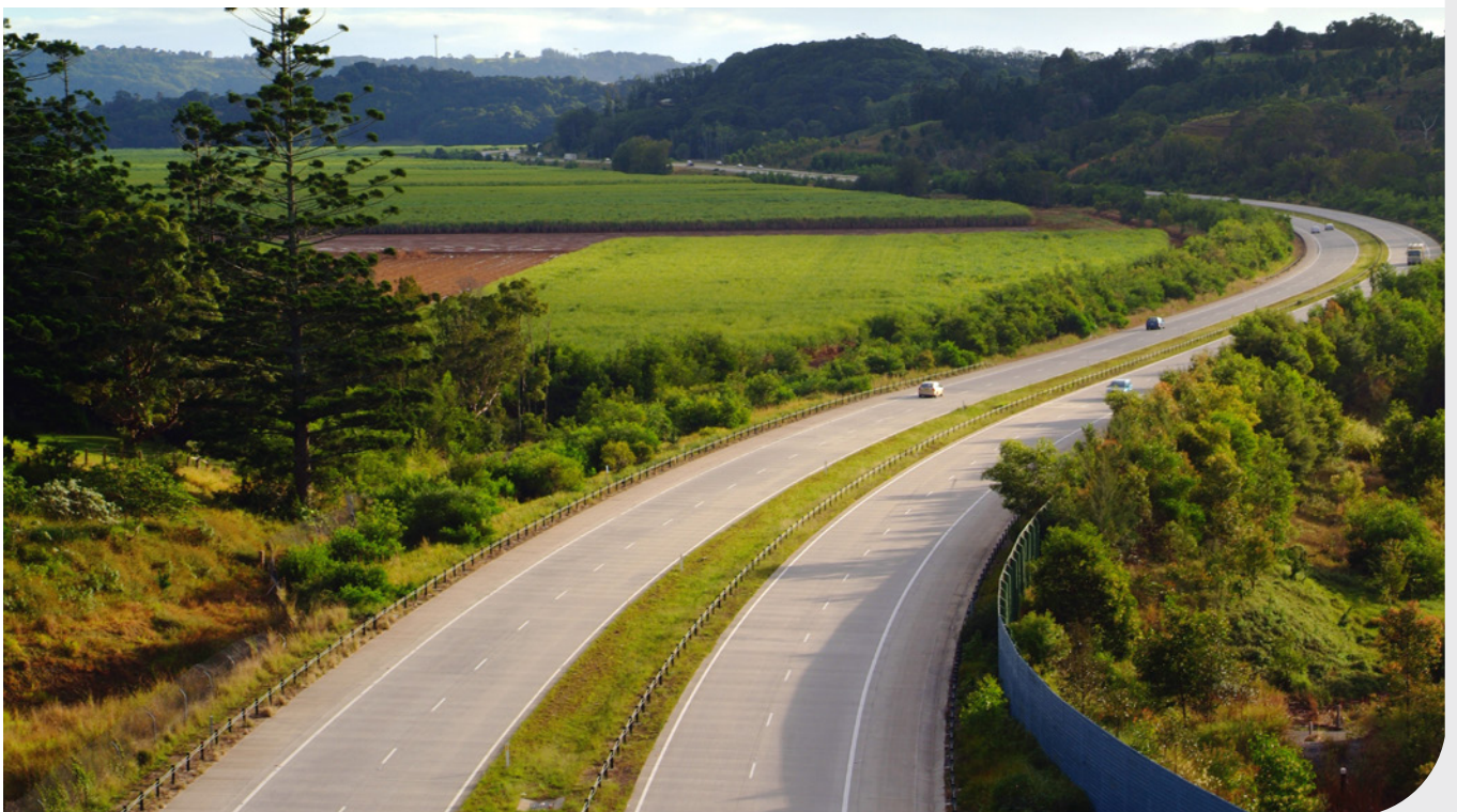
Yelgen to Chinderah Motorway.
