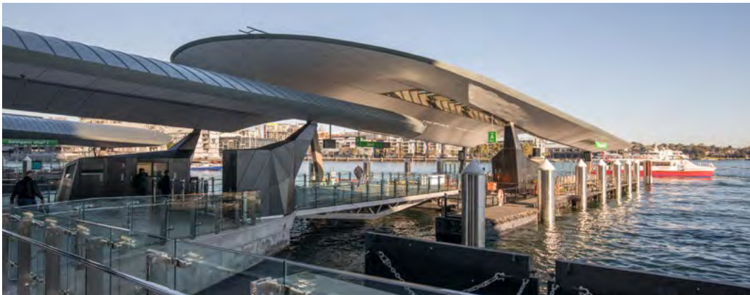
Barangaroo Ferry Wharf
