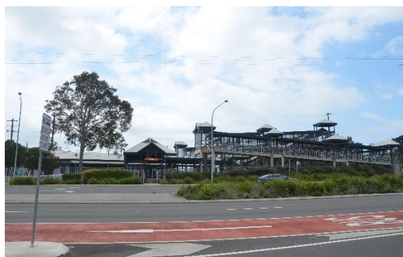
FIGURE 5-4 TUGGERAH STATION WESTERN ENTRANCE, THE PACIFIC HIGHWAY
