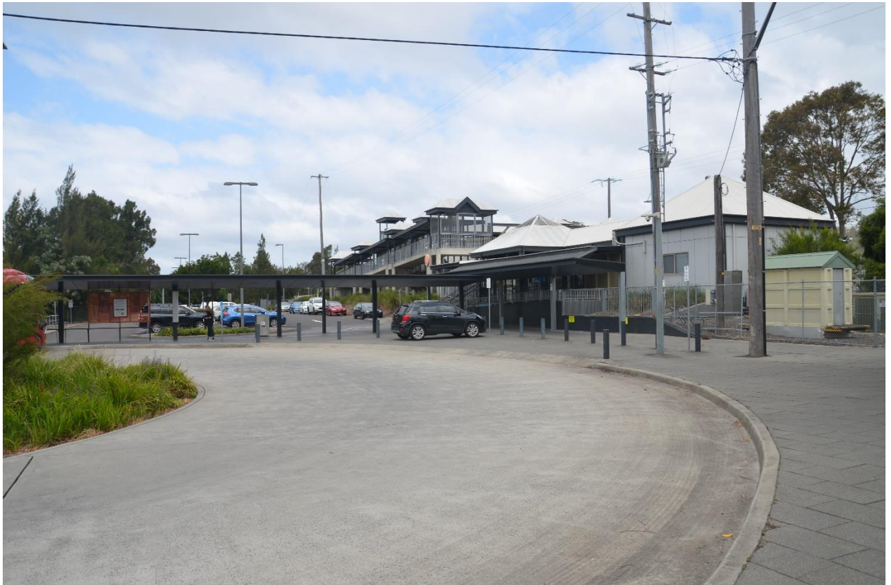
FIGURE 5-12 VIEWPOINT 4: VIEW SOUTHWEST FROM THE BUS INTERCHANGE
