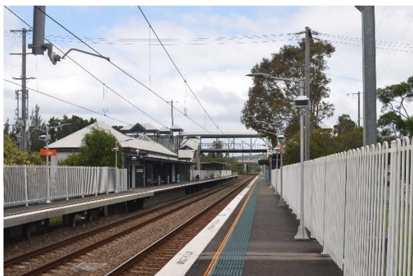
FIGURE 5-1 VIEW SOUTH ALONG THE TUGGERAH STATION PLATFORMS
