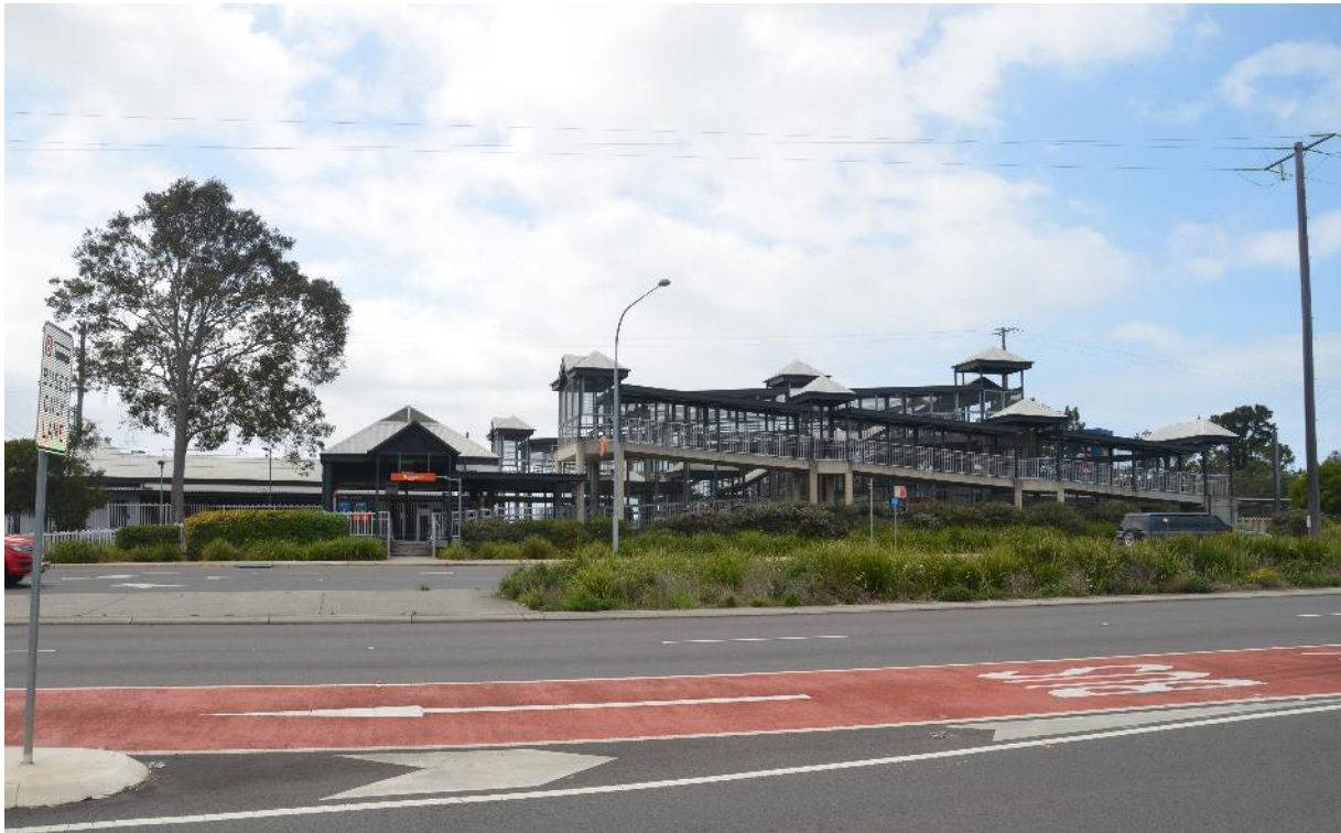
Figure 6-2 View of Tuggerah Station western entrance from the Pacific Highway
