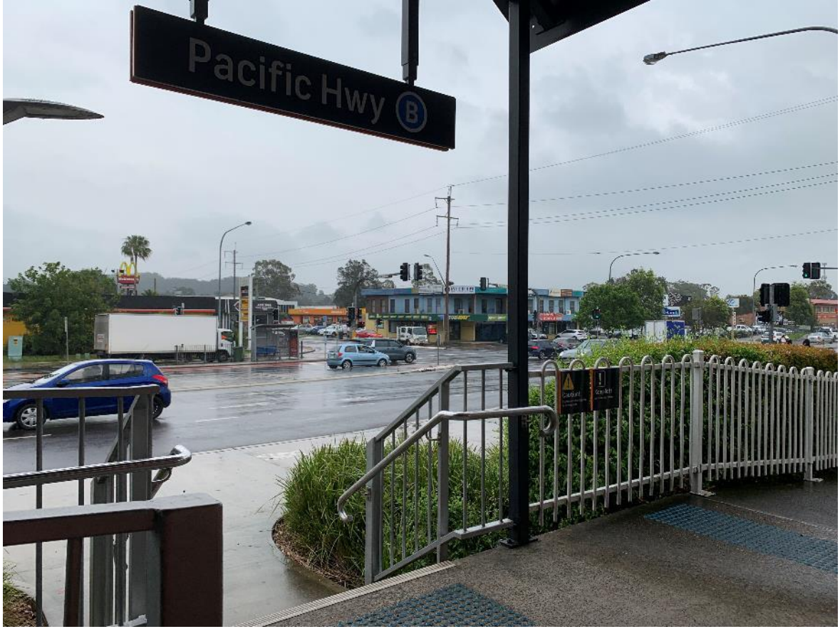
Figure 1-9 Pacific Highway station entrance, with existing signage, ramp and canopy
