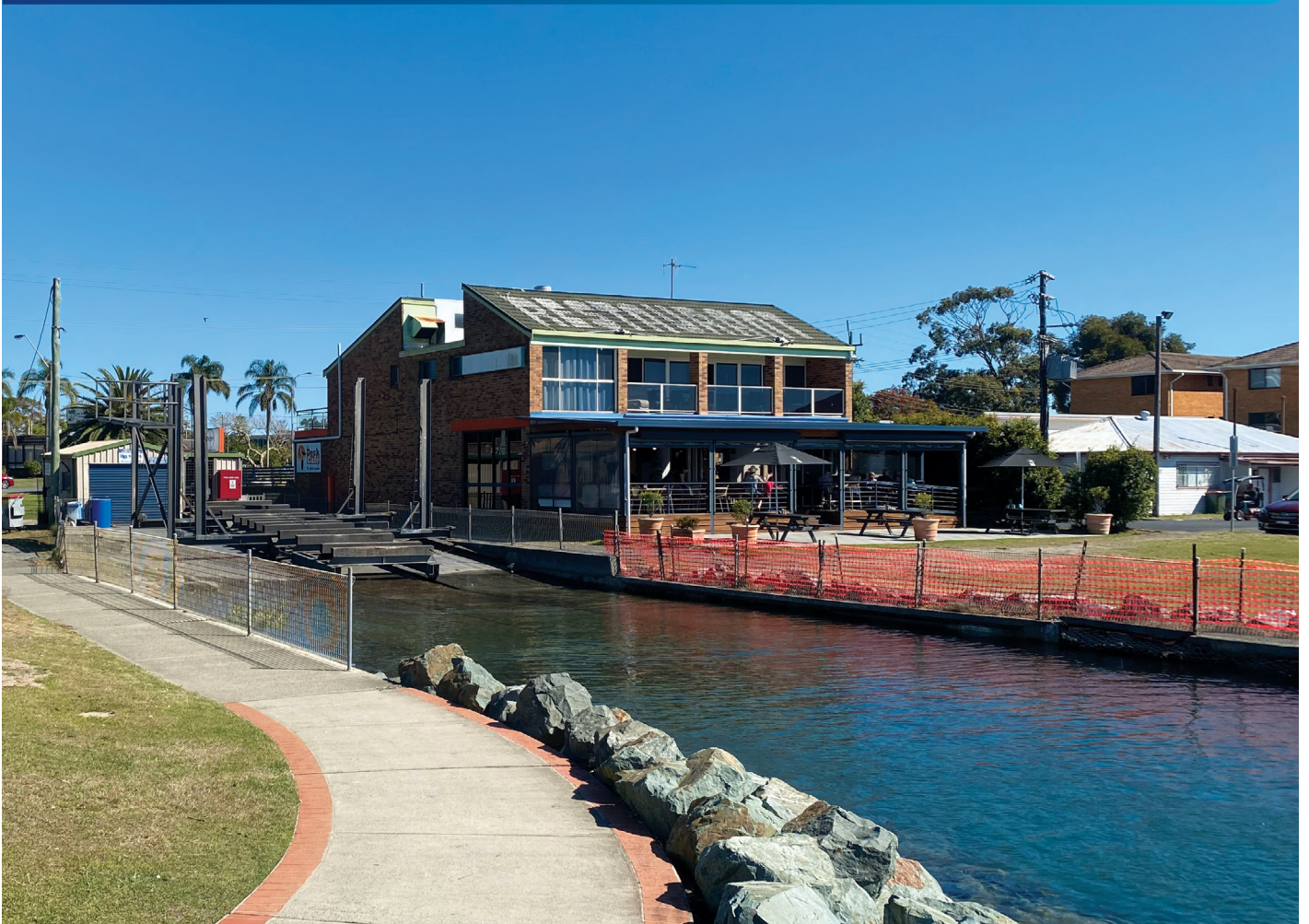
Tuncurry Boat Maintenance upgrade (current slipway)
