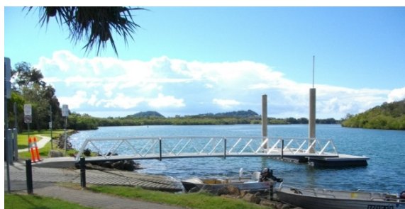
Lakes Drive Boat Ramp Upgrade & Pontoon, Tweed
