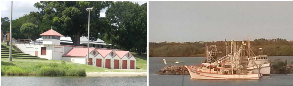
Figure 12 – Examples of rowing sheds for storage at Grafton, commercial fishing vessels stored at Yamba
