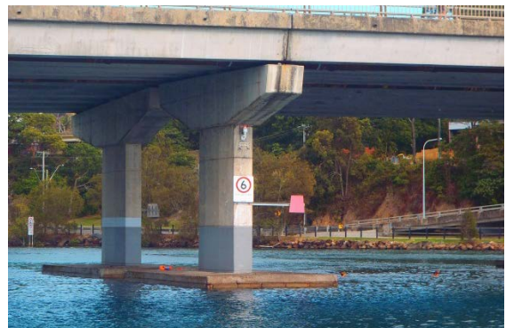
Multi-user area at Kennedy Road Bridge
