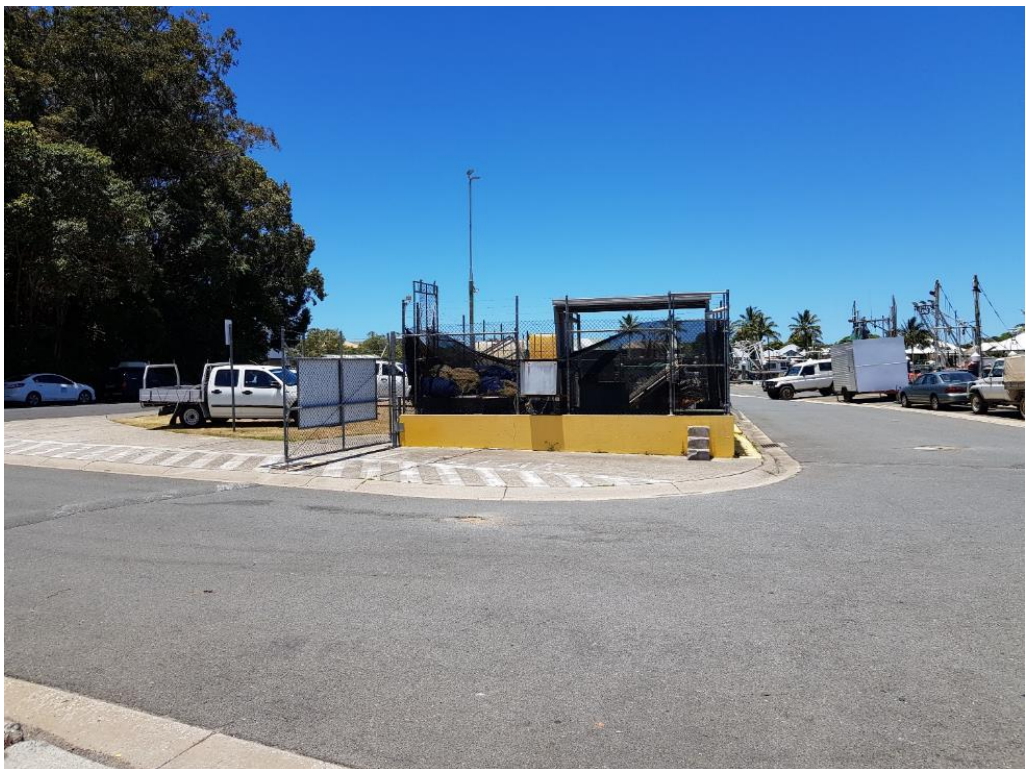
Figure 15: Existing entry way and storage yard
