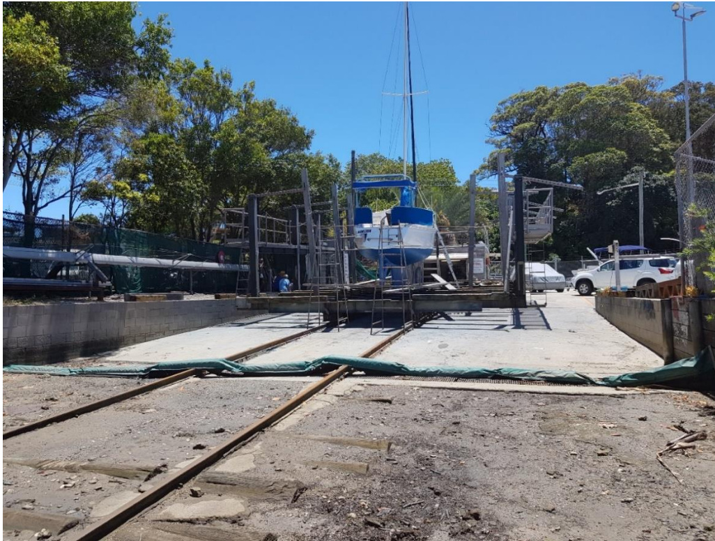
Figure 14: Existing boat ramp and slipway facility with the maintenance shed and car parking in the background
