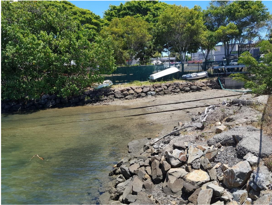
Figure 12: Image facing downstream across the existing boat ramp and slipway facility
