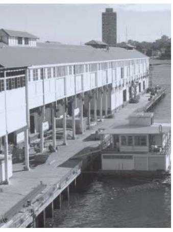
The refurbishment of Walsh Bay Pier 2/3 continued during the year and comprised replacement of worn piles and substructure as well as the roof and wall cladding
