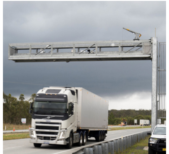
Figure 6: An example of an average speed camera in NSW. Copyright State of New South Wales (Transport for NSW)
