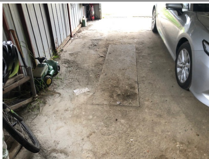
Photograph 6: Sediment accumulating in the detached garage is possible evidence of erosion near the rail corridor boundary.
