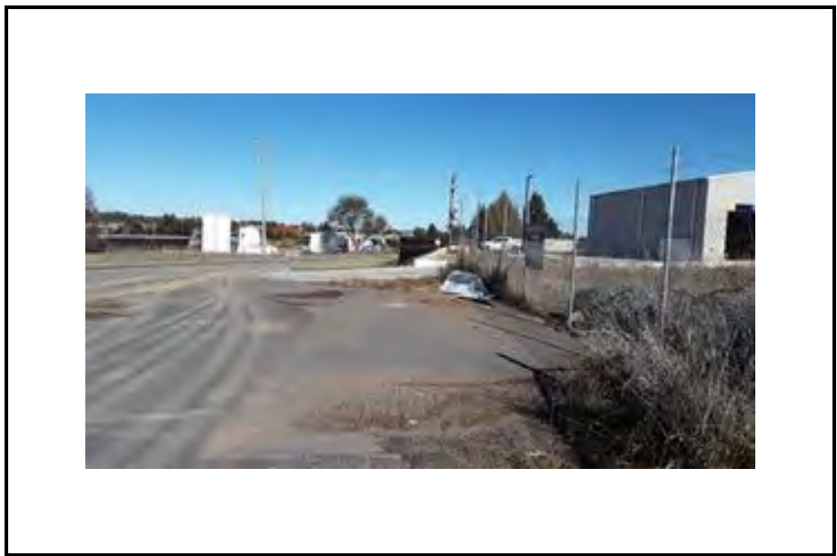
Photo 28: Photograph of heavily concreted area of working construction site at sample location XS211
