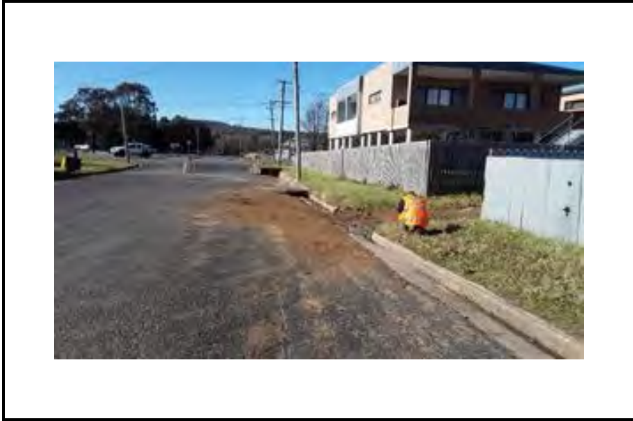
Photo 17: Sampling location XS077. Large amount of sediment near drain and bare patches of grass near driveway. Suspected to be from car and foot traffic.
