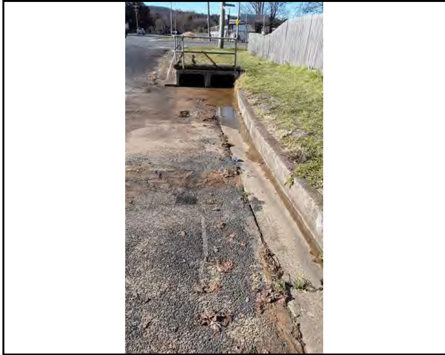
Photo 19: Photograph of drain and sediment on the South end of Ottiwell Street, corner of Ottiwell Street and Braidwood Rd.
