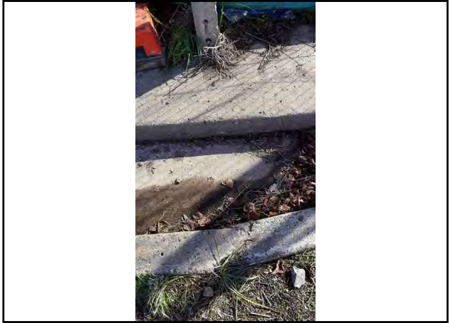
Photo 27: Photograph taken at sample XS211. Sample could not be taken due to asphalt pavement, concrete gutter and a high fence on concrete for construction site.
