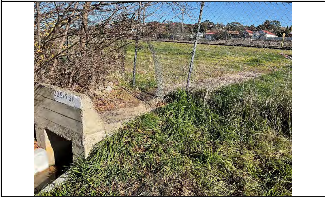
Photo 34: Drain on eastern end of Ottiwell Street on Wheat Yard boundary.
