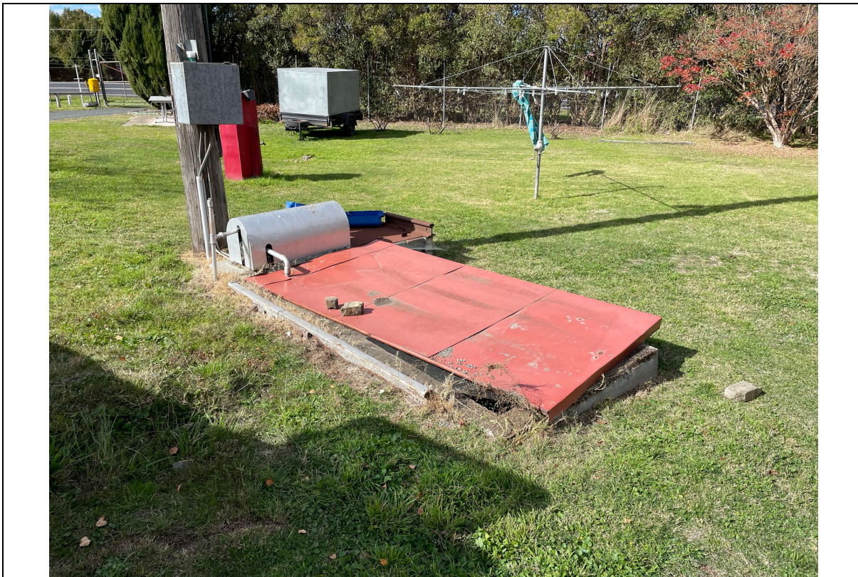
Photograph 23 View east towards surface water monitoring point SW01. .
