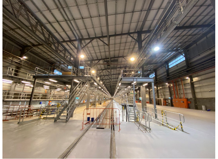
Train Maintenance Platforms inside the main facility
