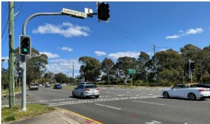
Image copyright The intersection of Princes Highway, Bates Drive and Garnet Road in Kareela.
