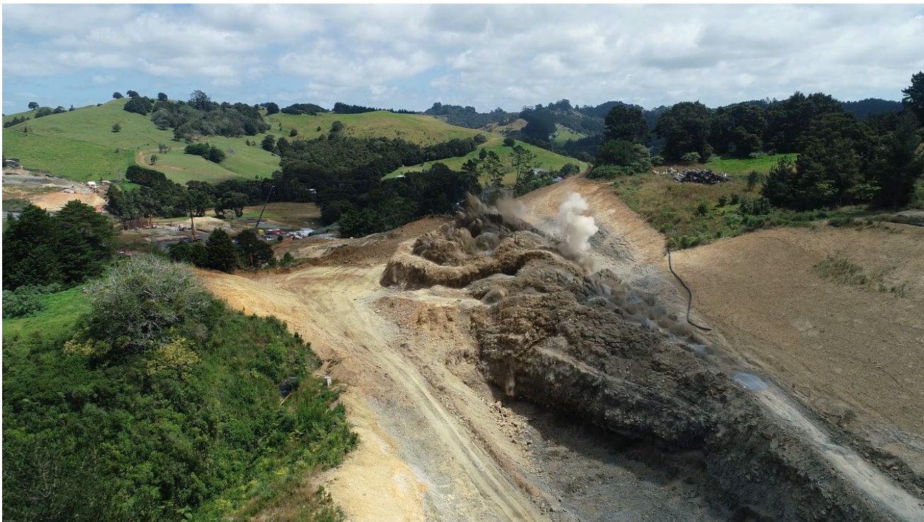
Controlled blasting at a cut site
