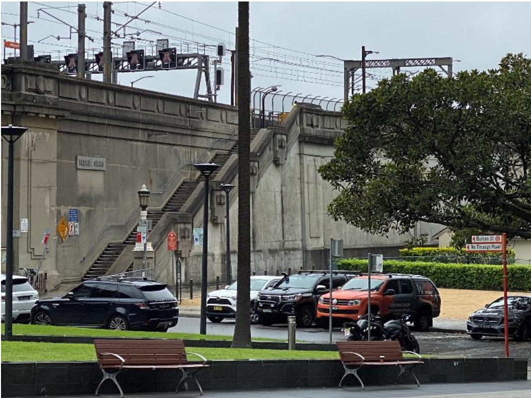
Figure 34: Northern approach for cyclists to the Sydney Harbour Bridge (Artefact, 2021)
