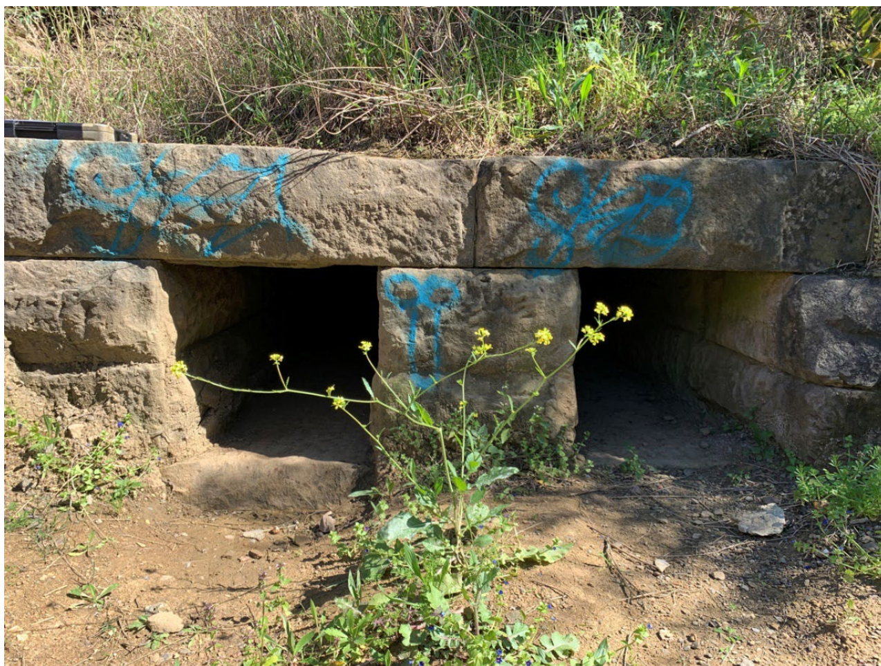
Photo 2.2 Sandstone box culvert located within the revised project area
