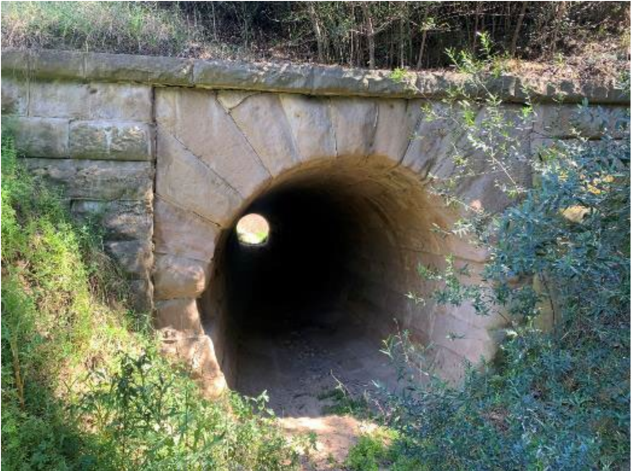
Photo 2.1 Sandstone arch culvert located within the revised project area
