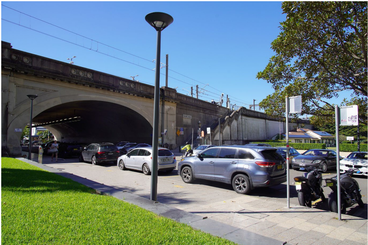
Figure 4-8 VIEWPOINT 9: VIEW EAST TO THE BURTON STREET TUNNEL ARCHWAY
