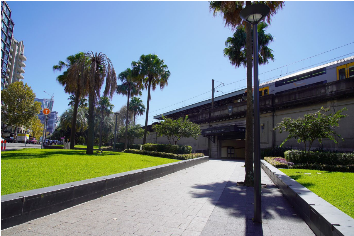
Figure 4-6 VIEWPOINT 8: VIEW NORTHEAST FROM BURTON STREET TO MILSONS POINT STATION FORECOURT AND ENTRANCE
