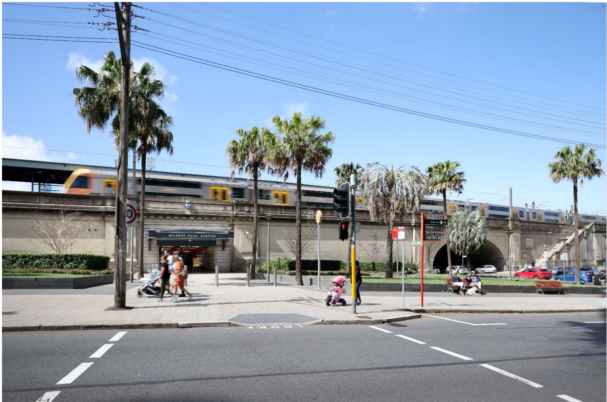
Figure 4-2 VIEWPOINT 4: VIEW EAST FROM ALFRED STREET SOUTH TO THE MILSONS POINT STATION ENTRY
