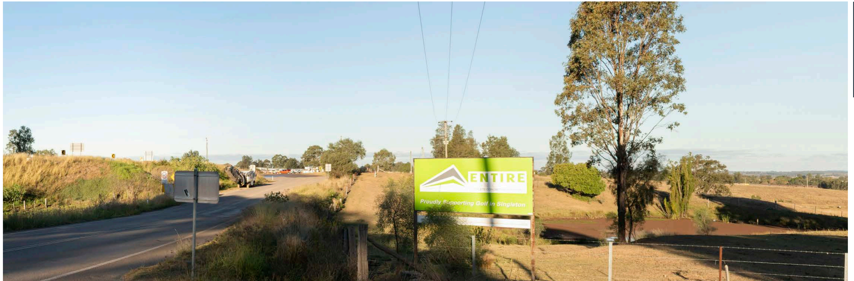
Figure 117: Zoomed-in current View of Maison Dieu Road Intersection
