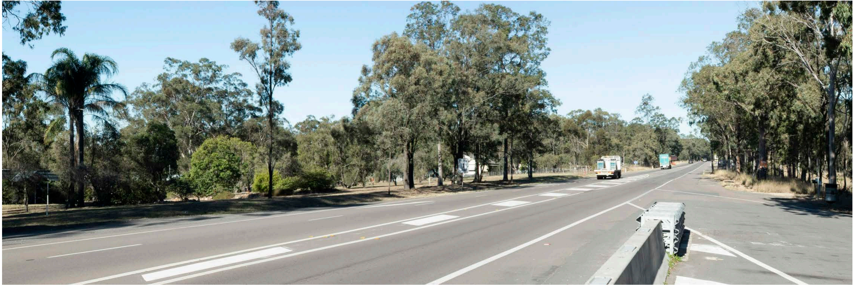
Figure 109: Zoomed-in current View of New England Highway South
