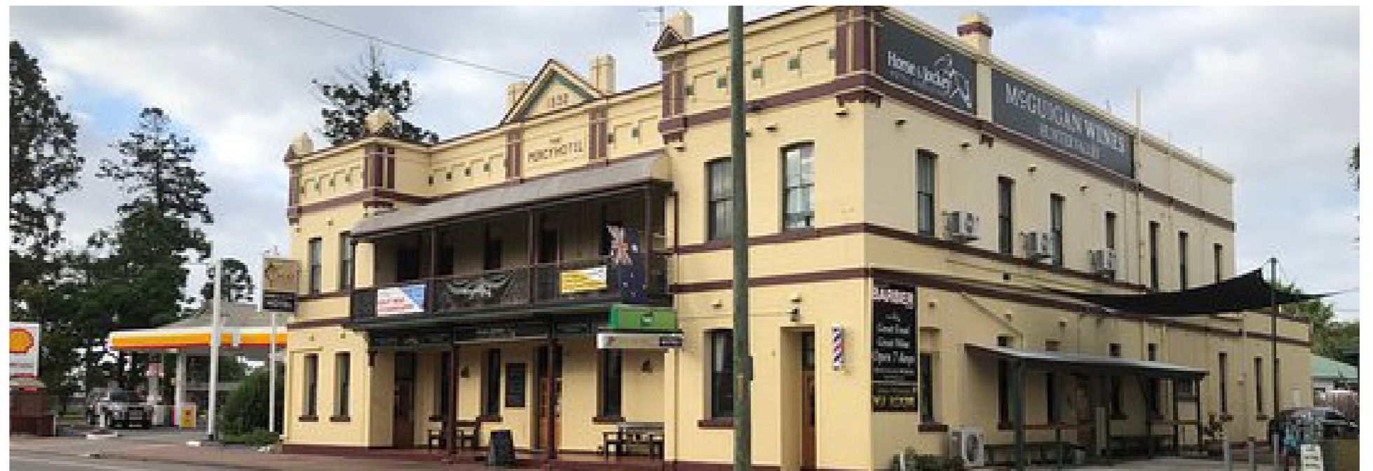
Figure 35: The Percy Hotel on George Street in Singleton Old Town (Source: Google Images)
