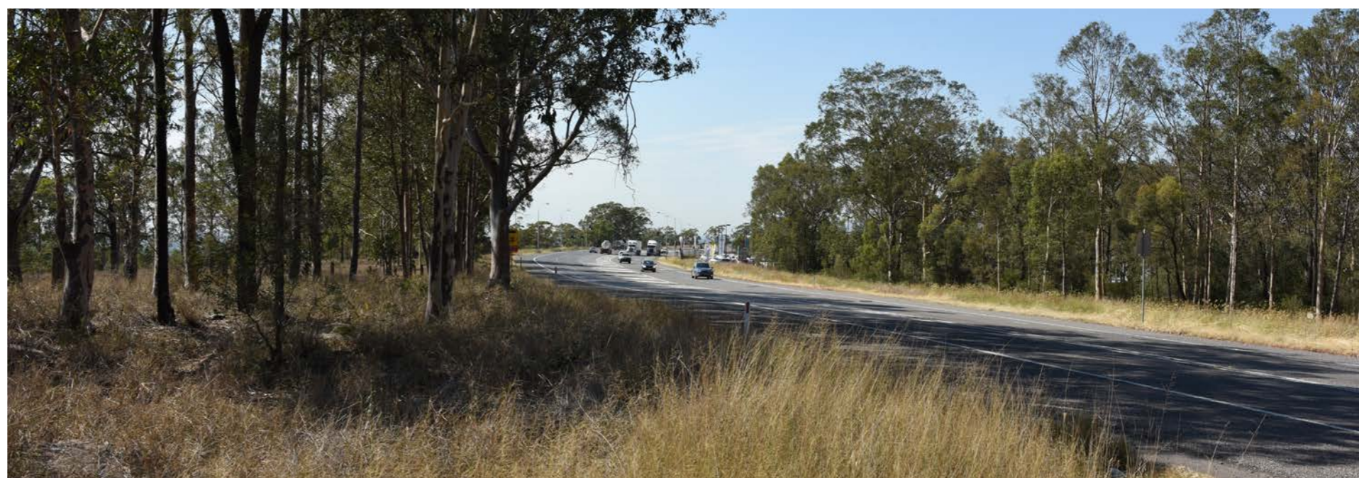
Figure 23: View looking south along New England Highway about 300 metres north of entry to McDougalls Hill Industrial Estate
