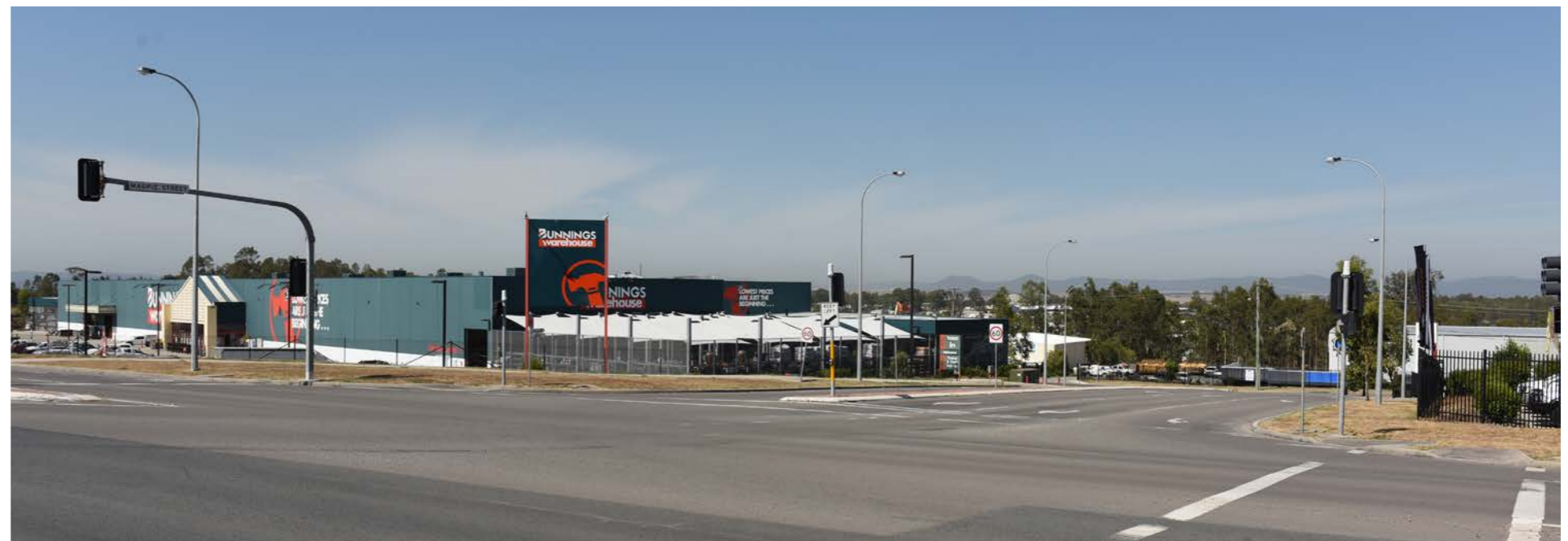
Figure 28: View of Magpie Street entry to McDougalls Hill Industrial Estate near the high point, with the Greater Blue Mountains World Heritage Area seen on the horizon
