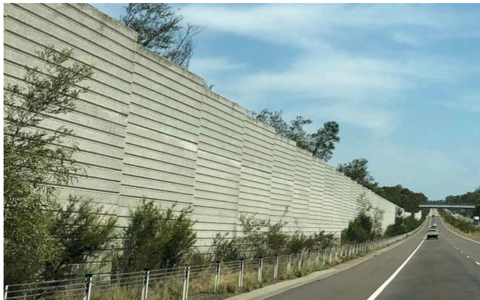
Figure 77: Typical noise wall arrangement from Hunter Expressway to be considered for Noise Wall Type 3
