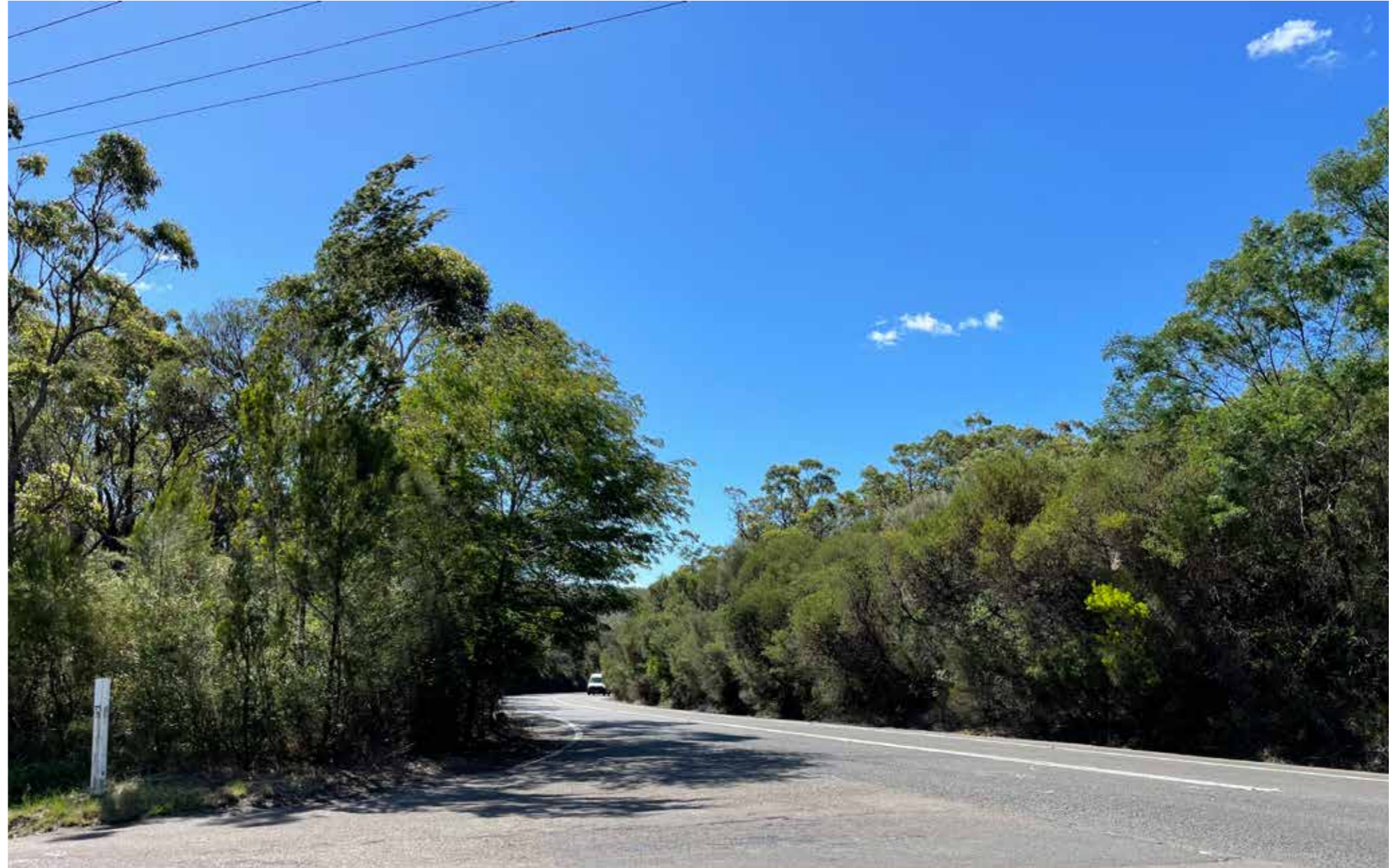
VP10 - Northbound view of Wakehurst Parkway just north of Oxford Falls Road
