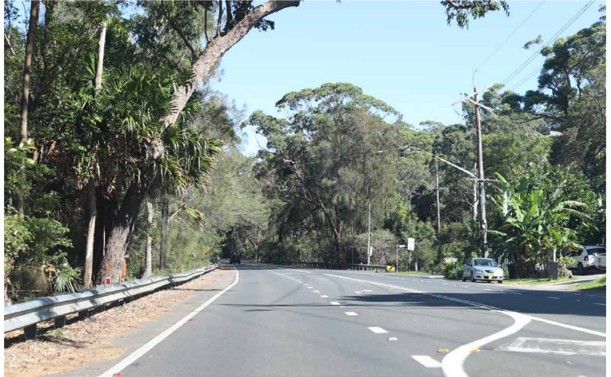
VP01 - Wakehurst Parkway westbound carriageway at Elanora Road
