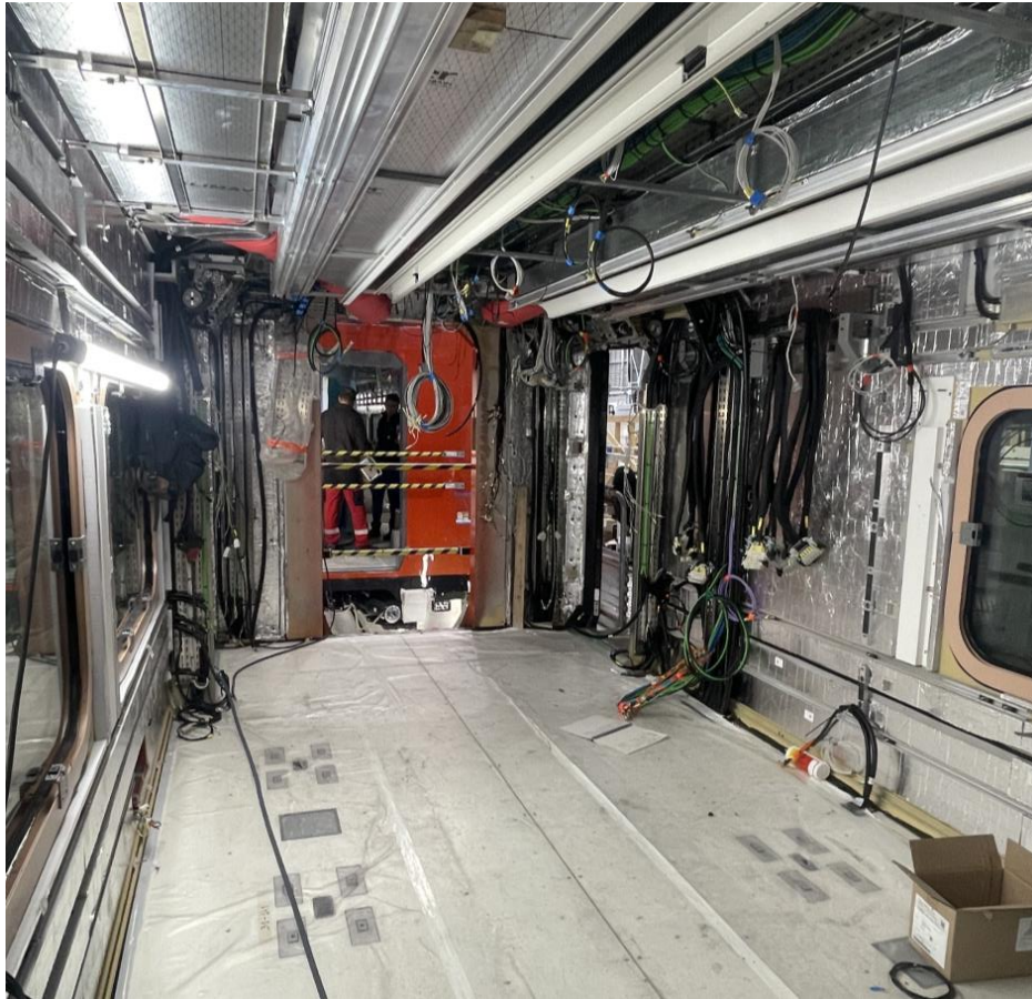
LR02 undergoing wiring fit out
