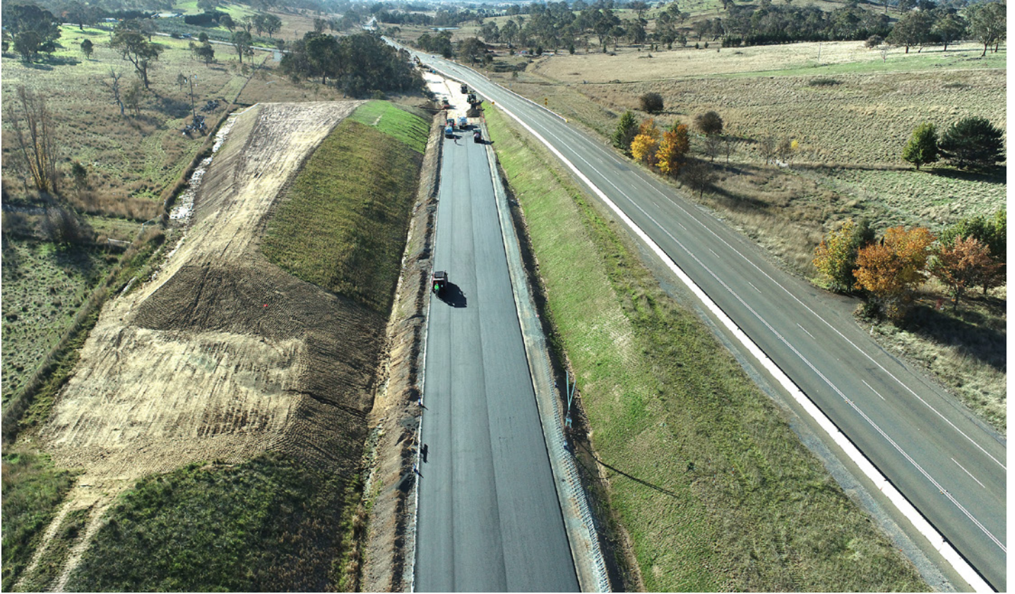
Seven kilometres of duplication has been completed on the Barton Highway.
