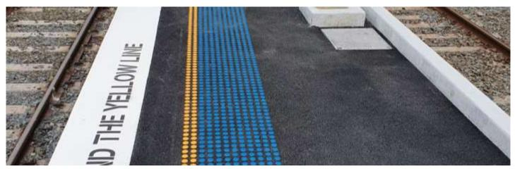
Section of platform extension including new asphalt, paint and tactiles at Kiama Station – August 2021
