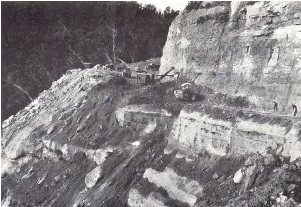
Figure 8. Mount Tomah cutting in 1950, showing completed earthworks and base course laid. Source. Department of Main Roads.
