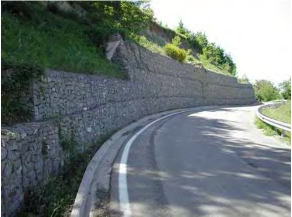
Figure 6-26: Example of a gabion wall
