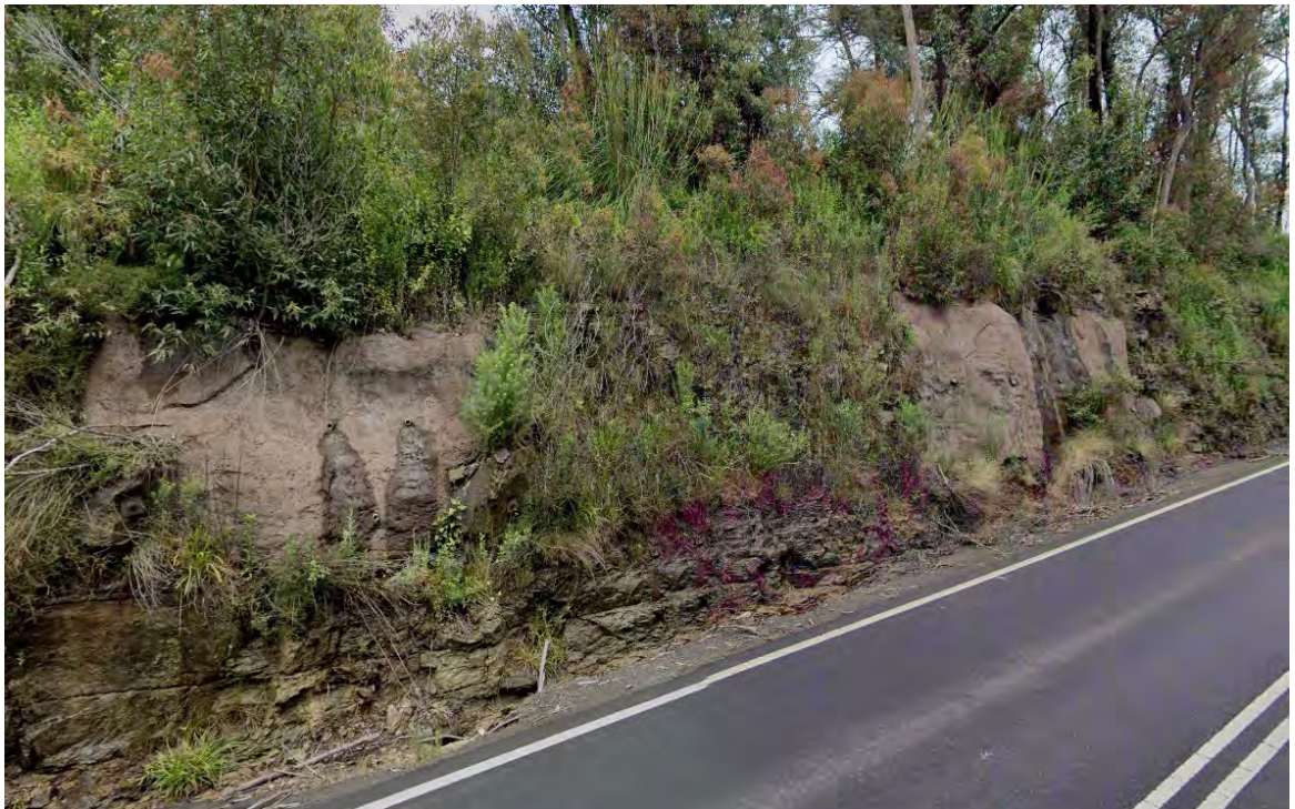
Figure 6-27: Example of existing shotcrete wall on Bells Line of Road
