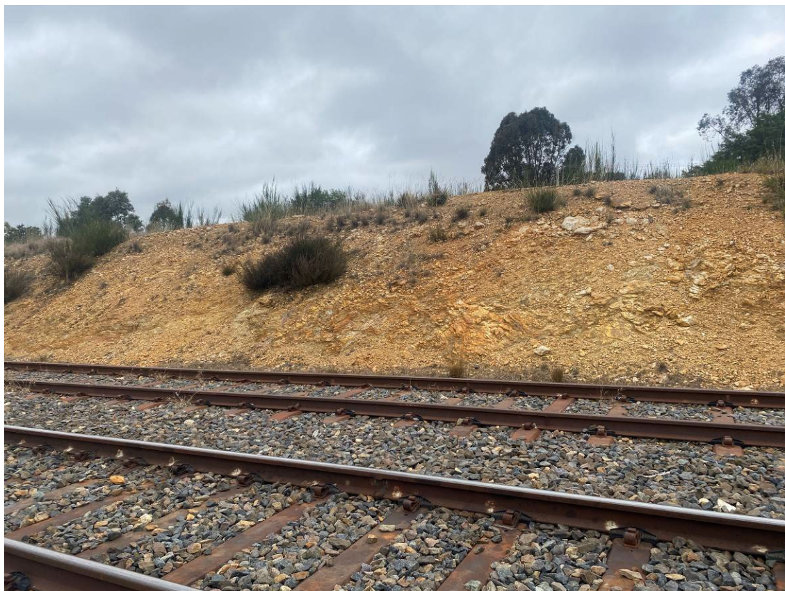
Photo 10: Evidence of erosion upgradient of train line facing east towards Powell Street. And opposite Station Master Cottage.
