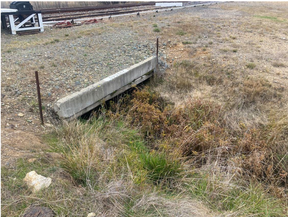
Photo 6: Downgradient of fourth culvert encountered on site from the south, near rail crossing on Malbon Street. Water slowly discharging through site. Clear and no turbidity after passing through weeds and reeds that act as natural sediment filters.
