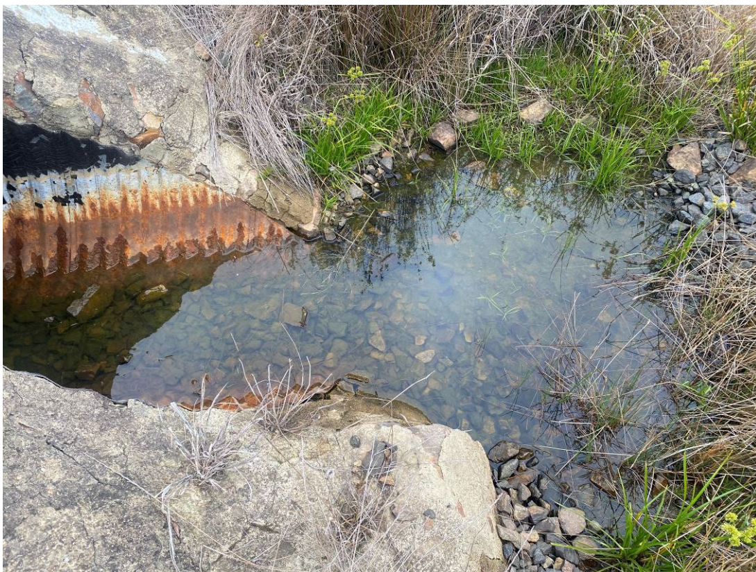
Photo 4: Downgradient of third culvert encountered on site from the south, discharges towards Majara Street, near King St intersection. Water pooled with no discharge of surface water off site. Clear and no turbidity.
