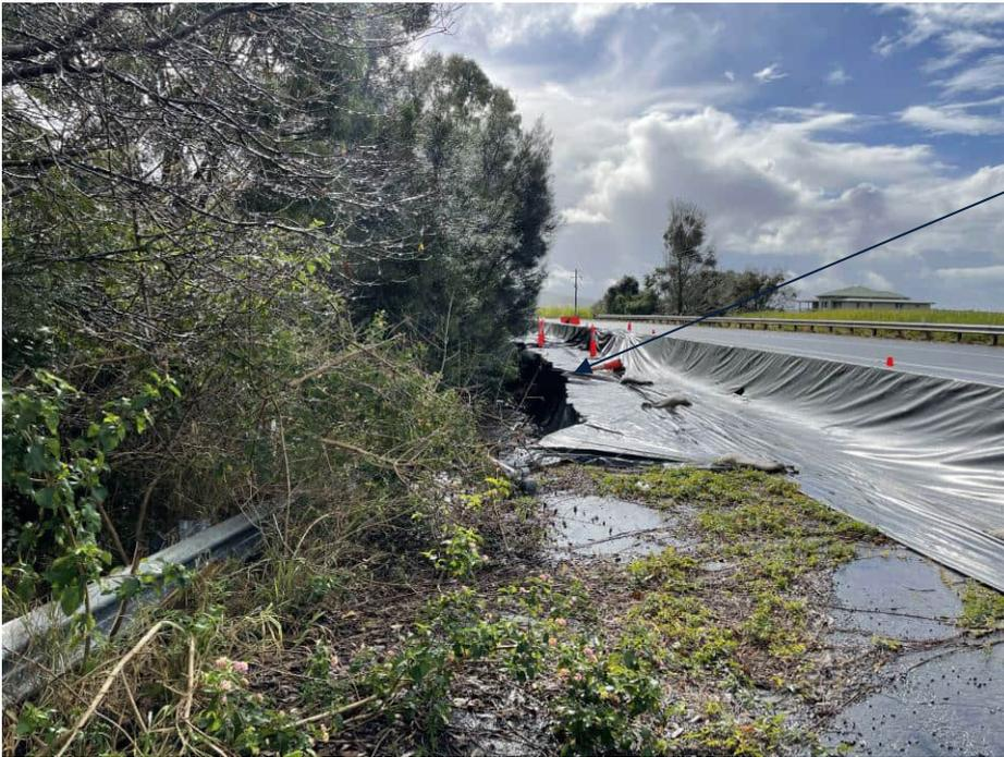
Slip headscarp with some slumping observed regressing back beneath pavement
