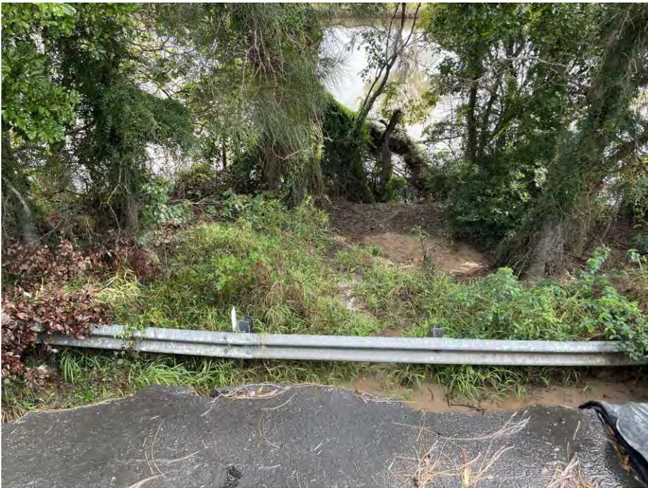
Photograph 4: ~Ch33515 – view of slumped road embankment and riverbank below headscarp.
