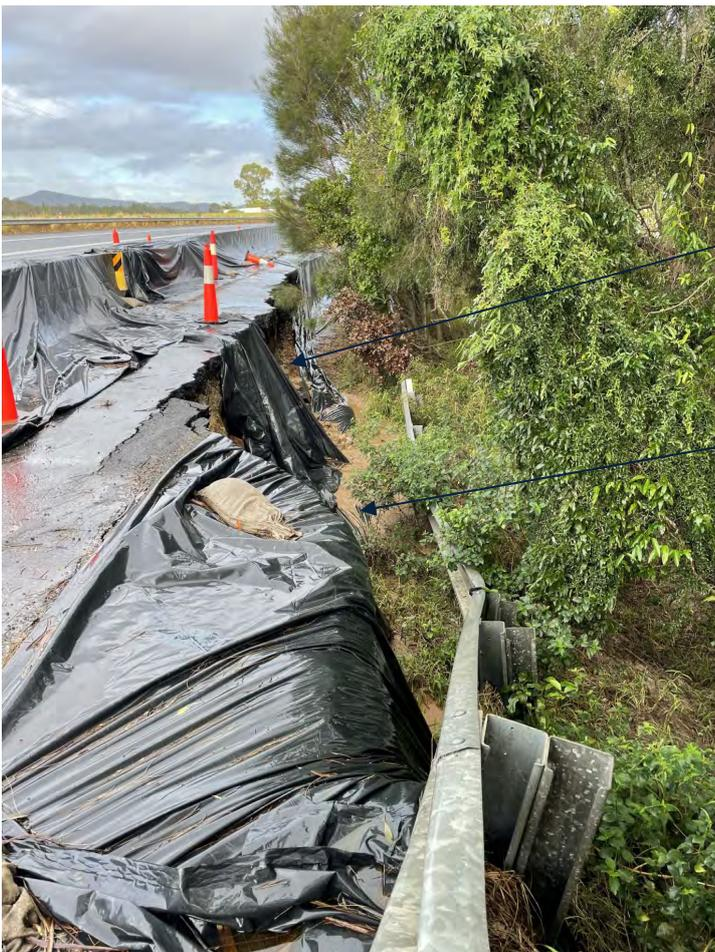
Recent slumping of headscarp pavement and fill materials. Regression back beneath pavement.
