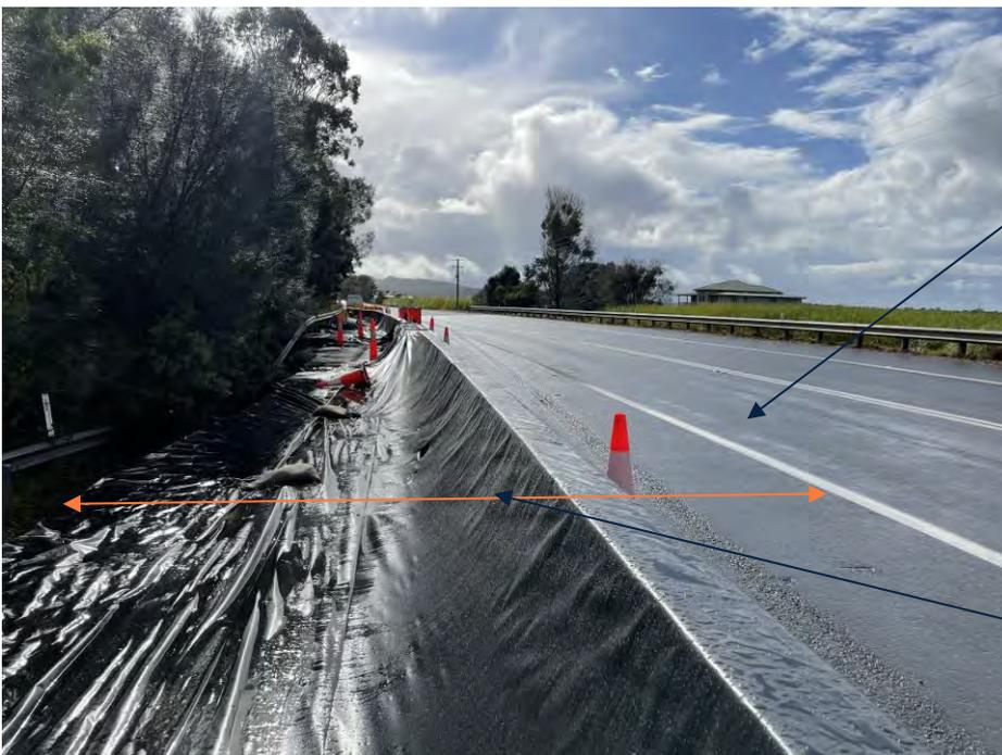
No obvious tension cracks observed in pavement. Pavement cross fall is towards the riverbank.
