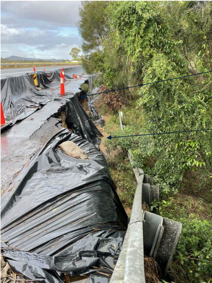
Slumping of headscarp pavement and fill materials. Regression back beneath pavement.
