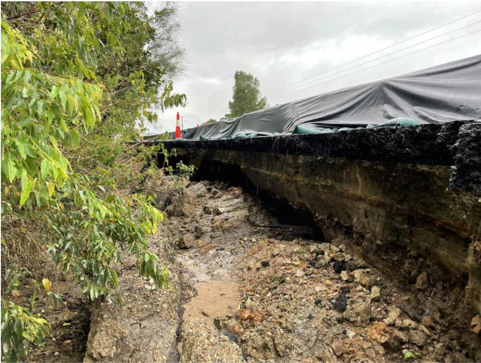
Photograph 3: 11 March 2021 - Headscarp exposing pavement layers and undercutting.
