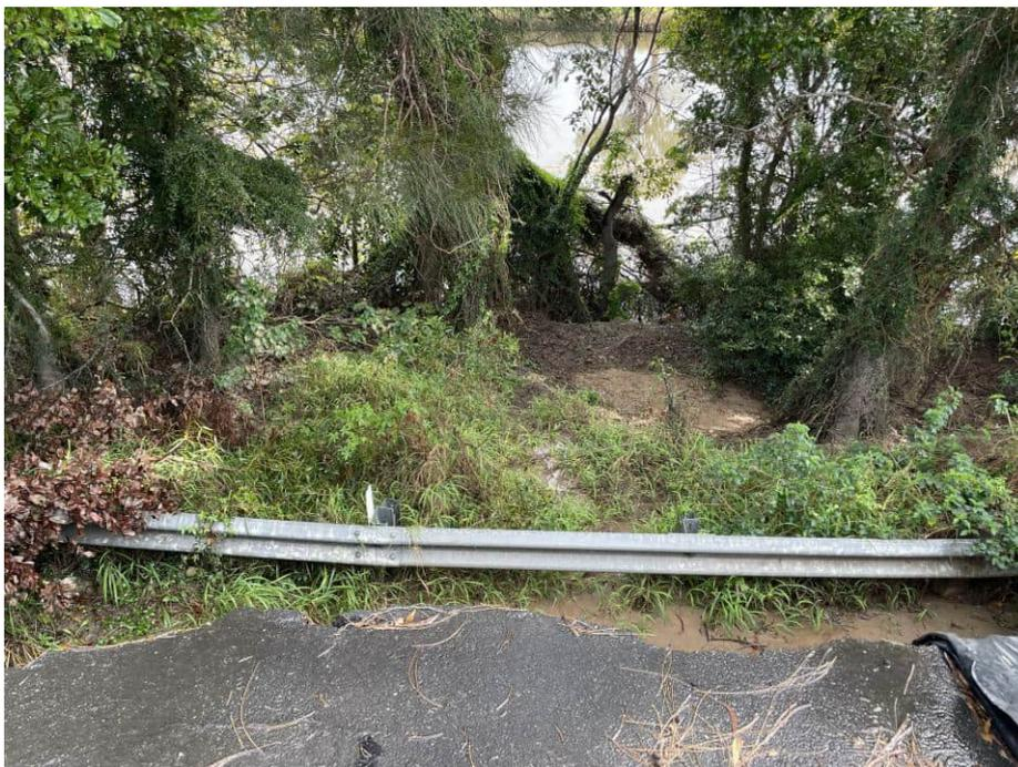
Photograph 8: 29 June 2021 - ~Ch33515 – view of slumped road embankment and riverbank below headscarp.
