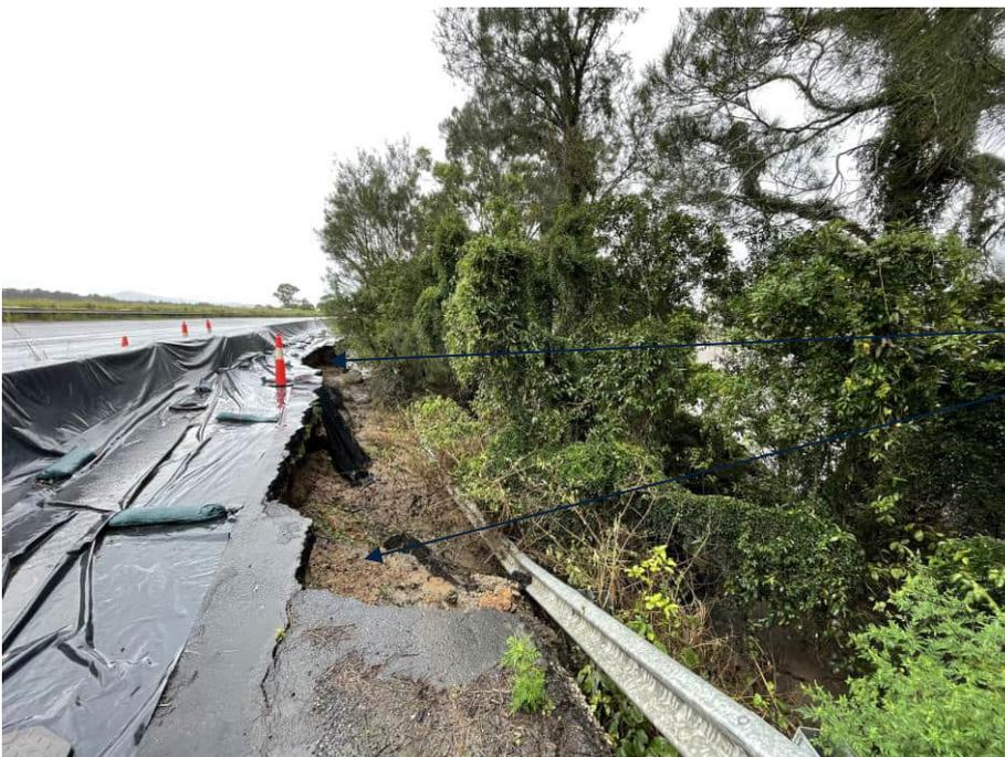
Additional slumping of pavement and fill materials. Regression back beneath pavement.
