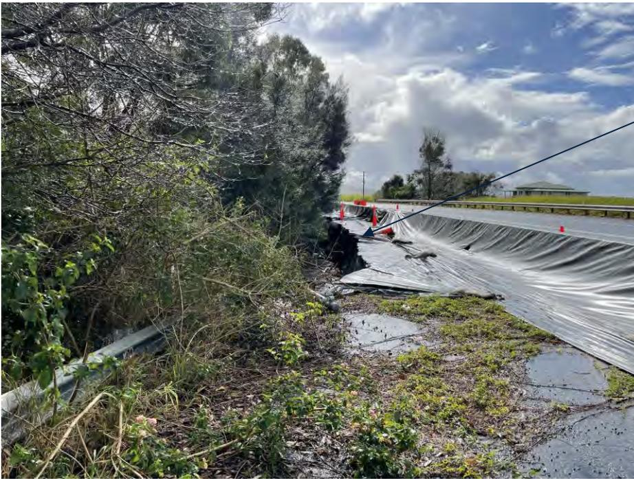
Landslip headscarp with some slumping observed regressing back beneath pavement
