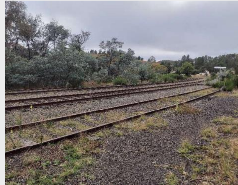
Rail corridor looking east
