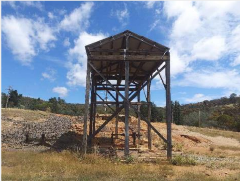
Former loadout facility
