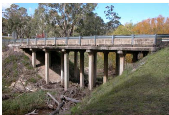
Surveyors Creek Walcha 1916 (RTA Bridge No 3485)
