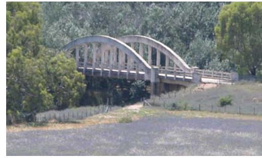
Hillas Creek Bridge on old Hume Highway, Tarcutta
