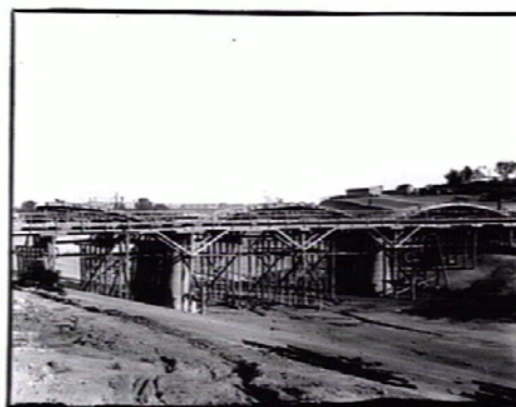
Monier arch construction, Victoria. (Source: State Library of Victoria)
