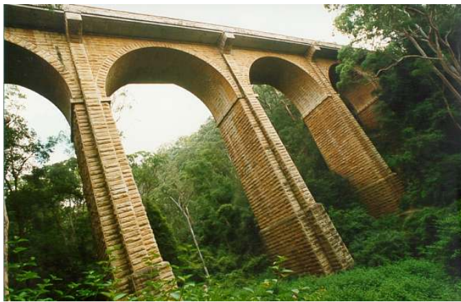
Lapstone masonry arch bridge (Photo NPB Photographics)
