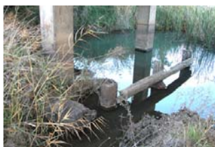
Previous pier timbers, Tyagong
