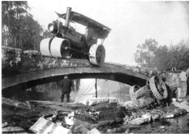
Kings Bridge collapse during load test by steam and traction engines – both visible (source http://home.vicnet.net.au/~aholgate/jm/ )
