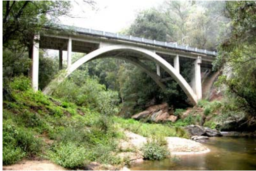
Bridge over Berowra Creek Galston (RTA Bridge No 389)
