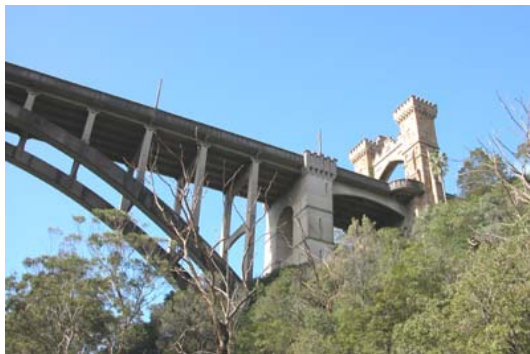
Northbridge southern abutment and tower (RTA Bridge No 172)
