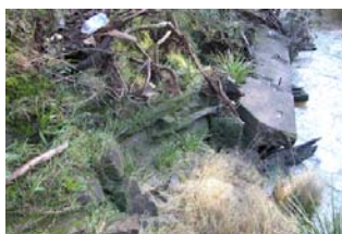
Old footing and headstock,
