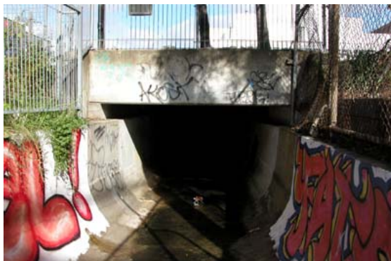
Entrance to culvert under Parramatta Road Burwood
