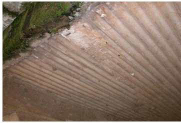
Corrugated iron formwork
