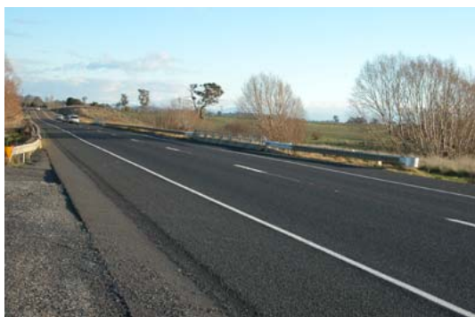
Jeir Creek Bridges 1 and 2 suggest little to the motorist
