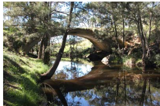
Oaky Creek Cobbadah (RTA Bridge No 3670)
