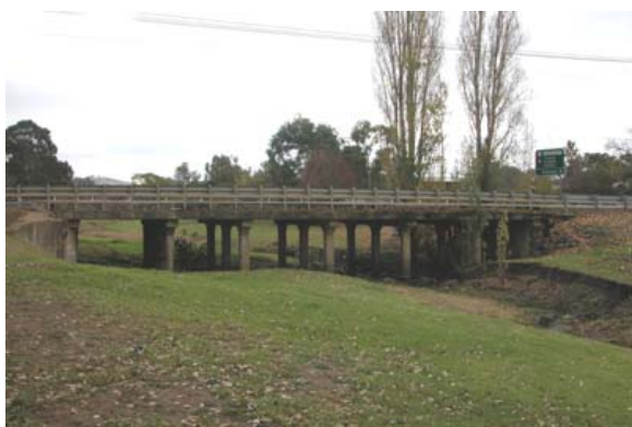
Muttama Creek Cootamundra 1914 (RTA Bridge No6438)
