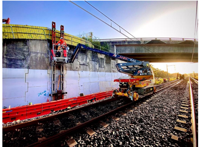
Works during scheduled rail shut down period in February 2023
